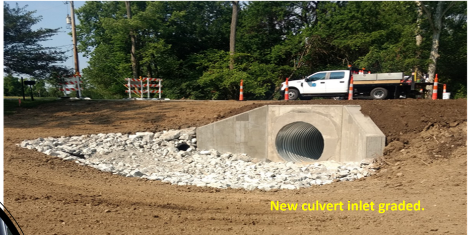
New culvert inlet with pre-cast headwalls.
