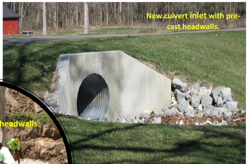
New culvert inlet graded.
