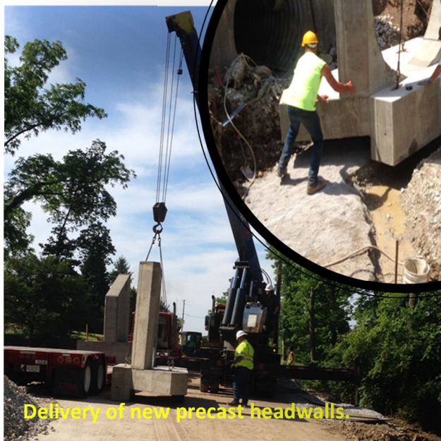
Setting new precast headwalls.
