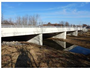
This bridge in Washington Township was posted for a reduction to legal load limits and supported by jacks due to deterioration of the abutments. The edges of the existing concrete slab had also deteriorated severely. Following the posting for a load limit, the County applied for a grant from the County Engineer's Association of Ohio
