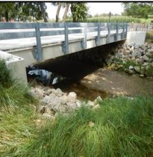
The Montgomery County Engineer's Office planned the reconstruction of the existing Chicken Bristle Road Bridge (JAC-60A-3.92) in Jackson Township over a tributary to Little Twin Creek. The existing single span bridge had poor deteriorated beams which placed the inspection rating of this bridge in fair condition. This bridge was built in 1968 and had well exceeded its life expectancy.
