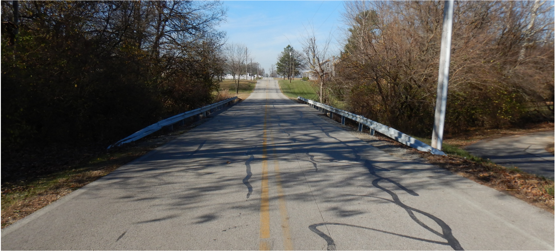
View of the bridge as seen from the East looking West
