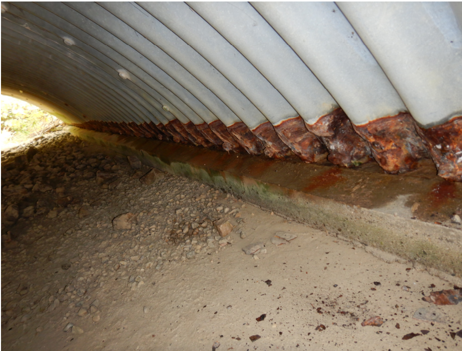
South Edge General Condition
