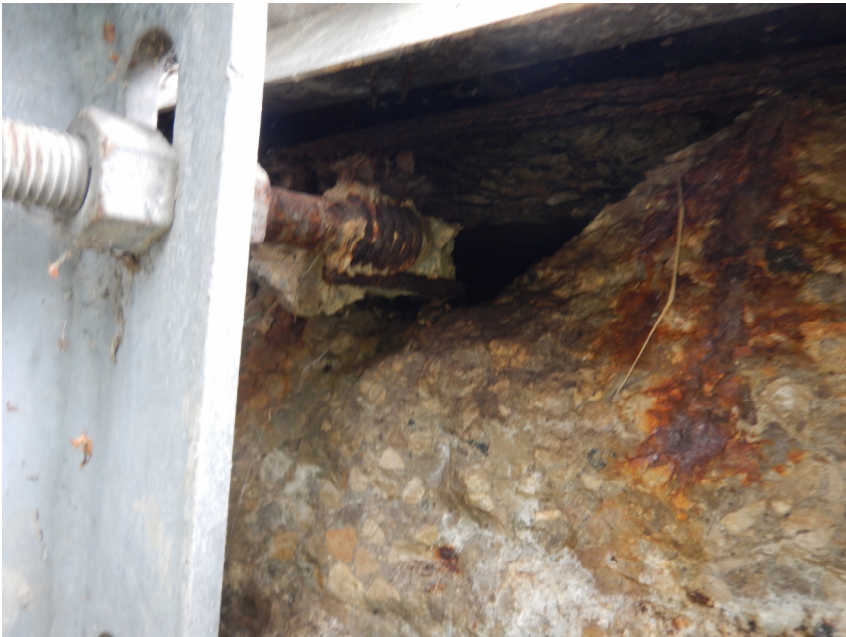
East Guardrail Connection
