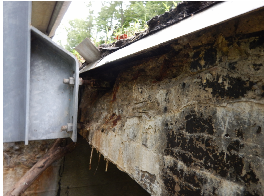
West Guardrail & Exterior Beam Spalling
