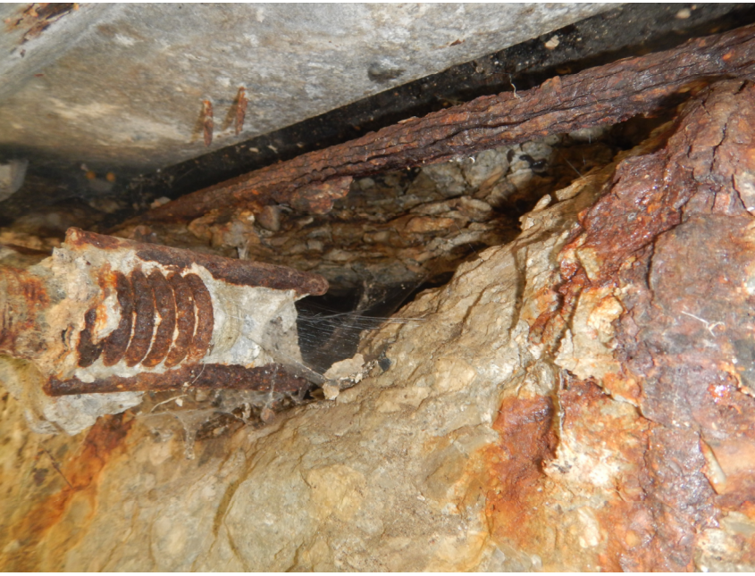
East Guardrail Connection
