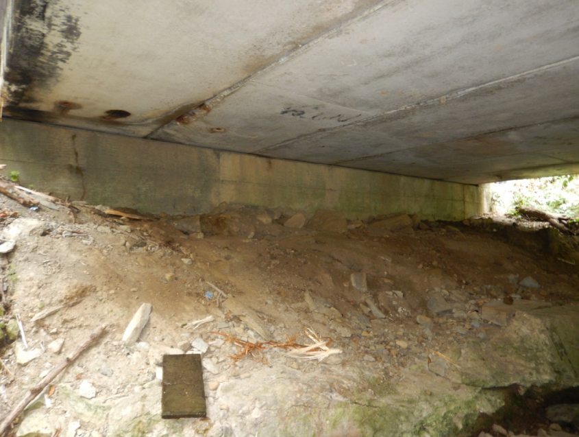
South Abutment & Beams
