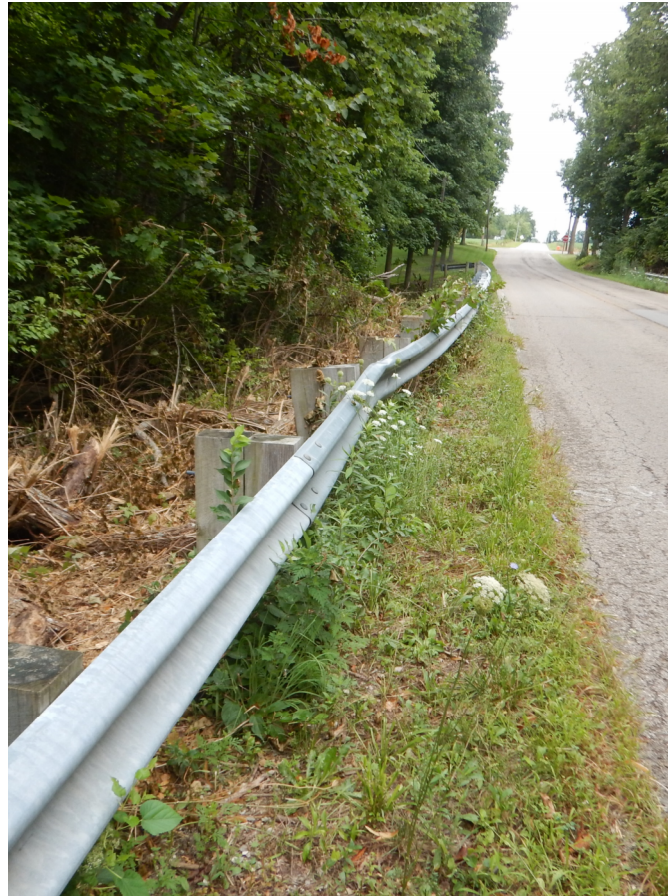
West Guardrail Looking North
