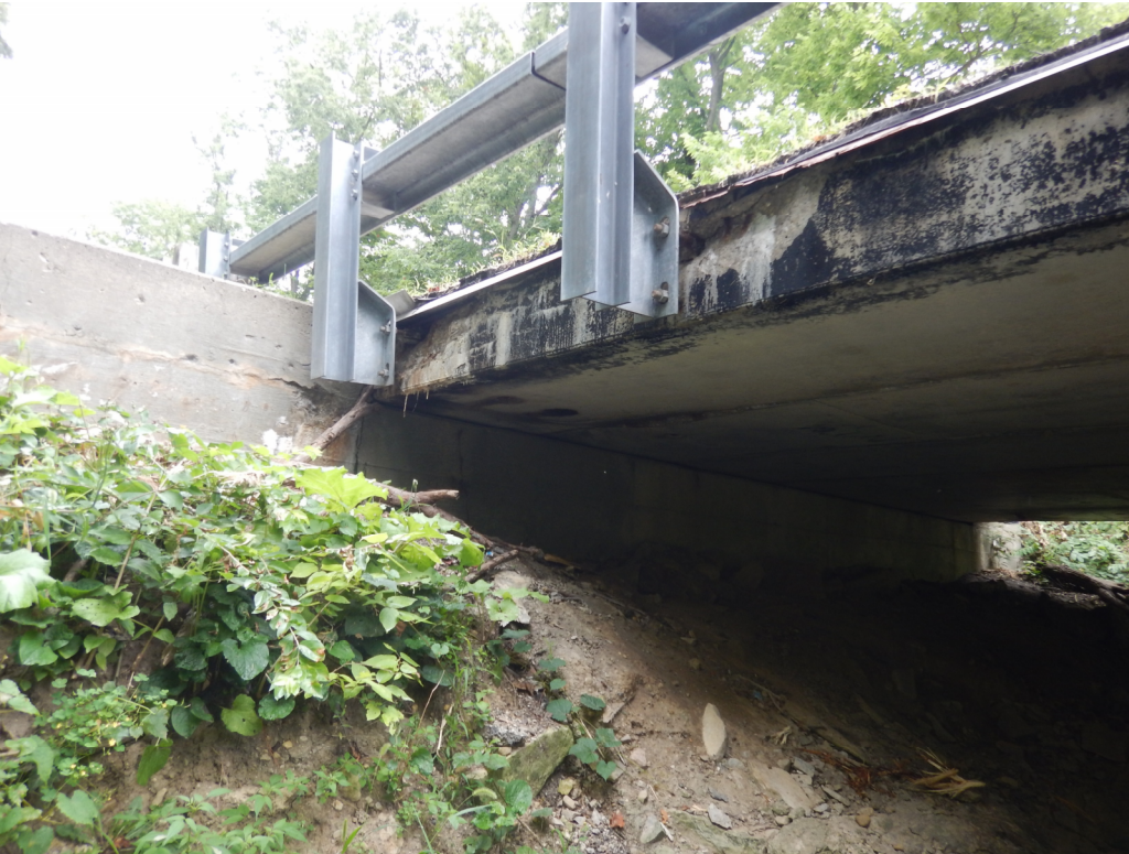
West Guardrail & Exterior Beam Spalling
