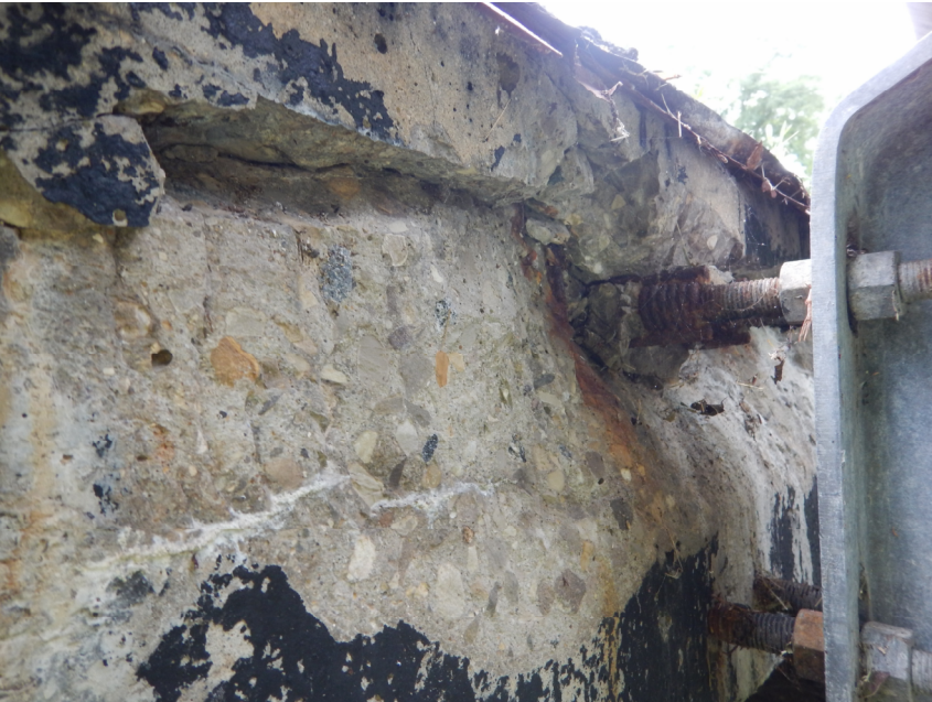
West Guardrail Connection
