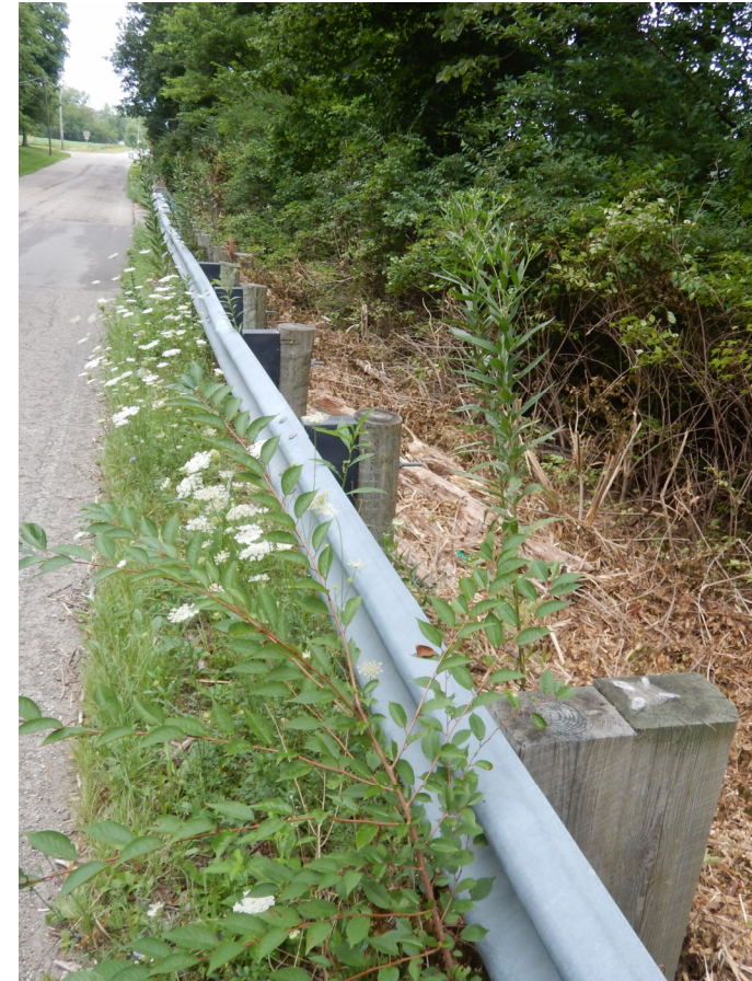
East Guardrail Looking North
