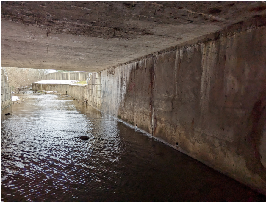
West Half of North Abutment Looking West
