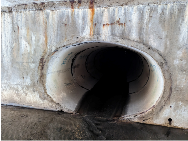
113" Span by 72" Rise" Elliptical Concrete Pipe Intersecting North Abutment Looking North
