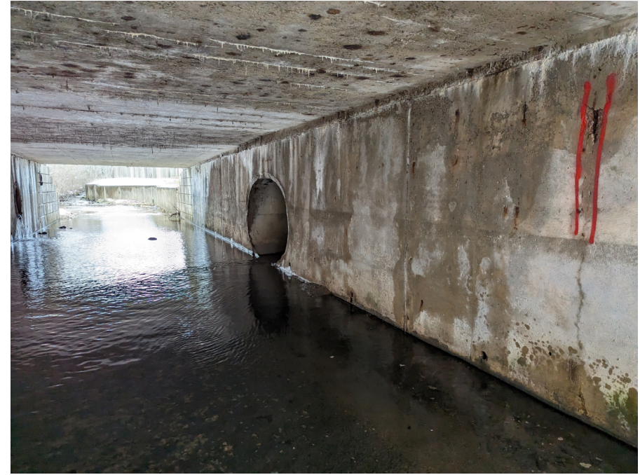
North Abutment Looking West
