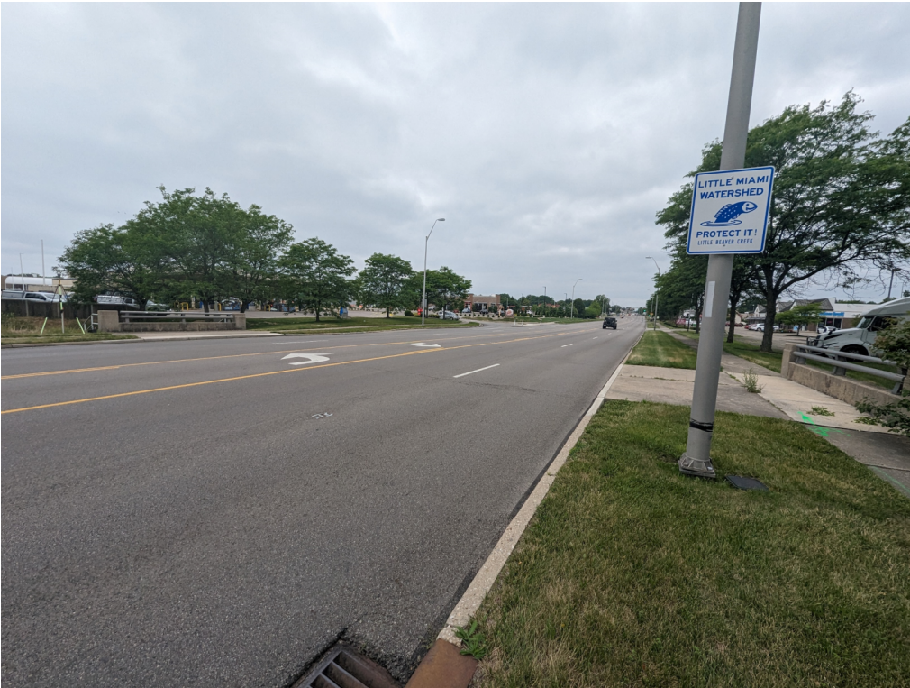
View of the Top of Wilmington Pike Bridge as seen from the Southeast Looking Northwest
