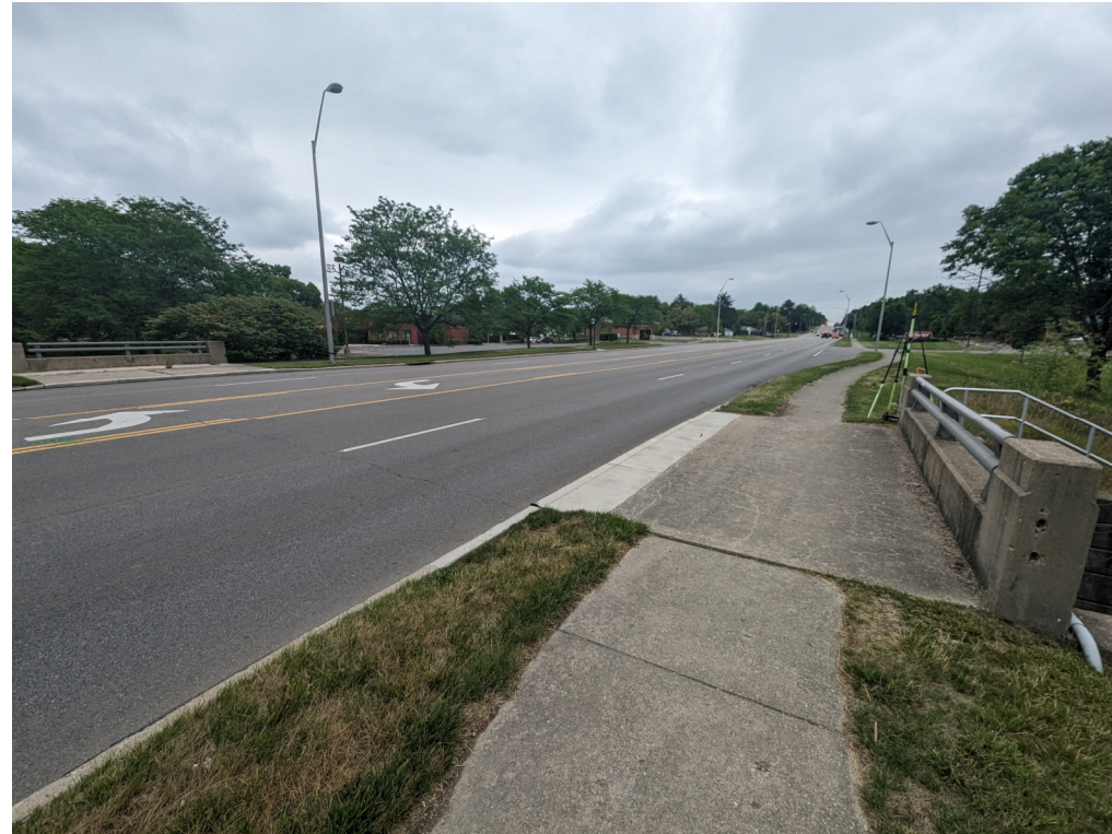
View of the Top of Wilmington Pike Bridge as seen from the Northwest Looking Southeast
