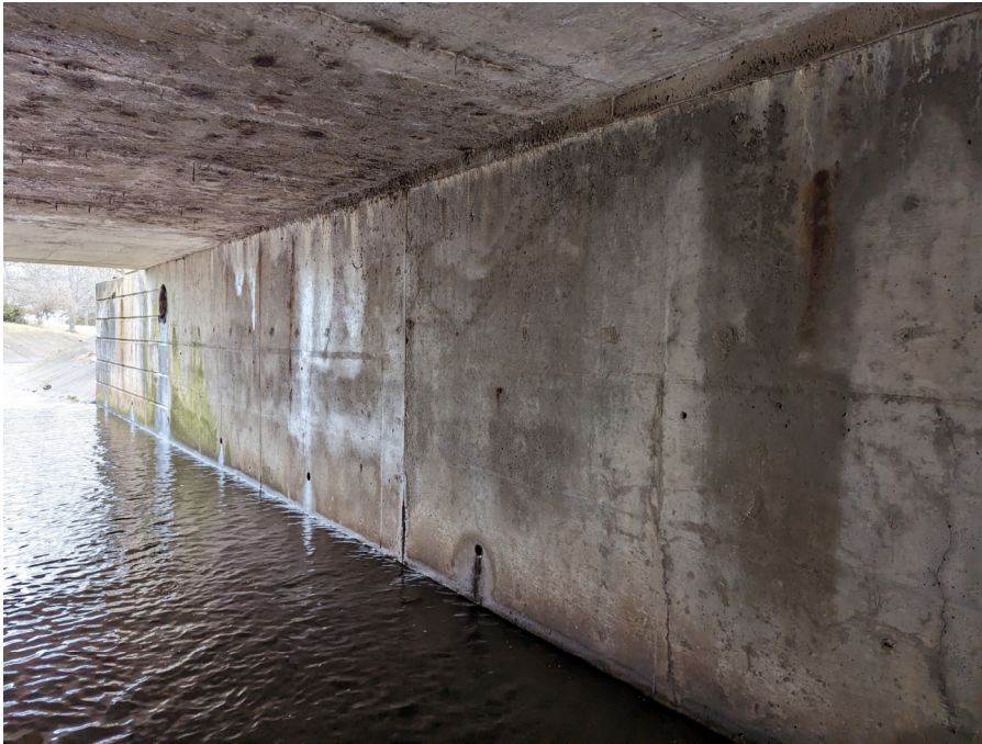
East Half of South Abutment Looking Southeast
