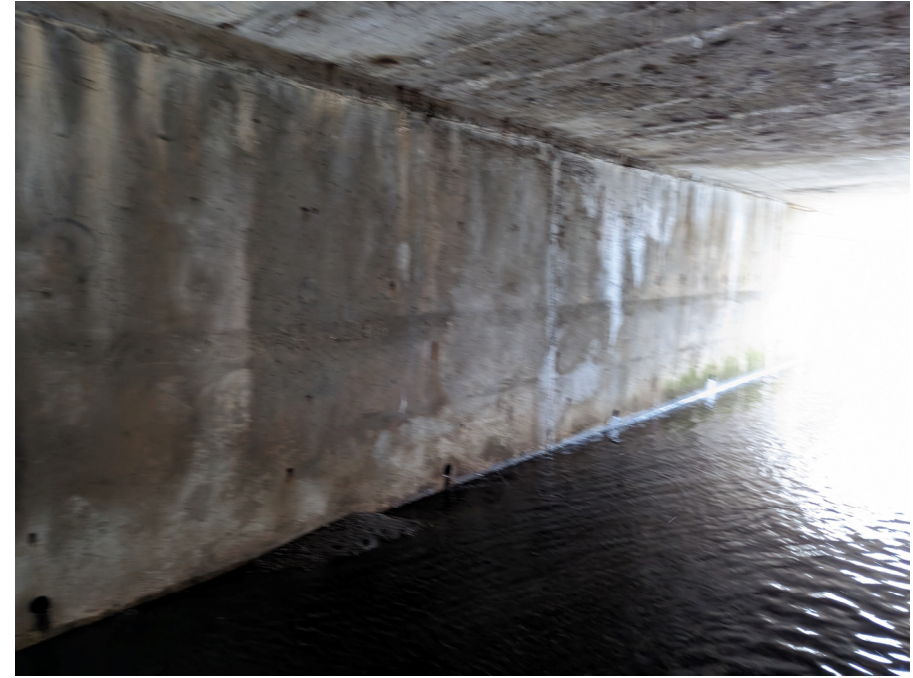
West Half of South Abutment Looking Southwest
