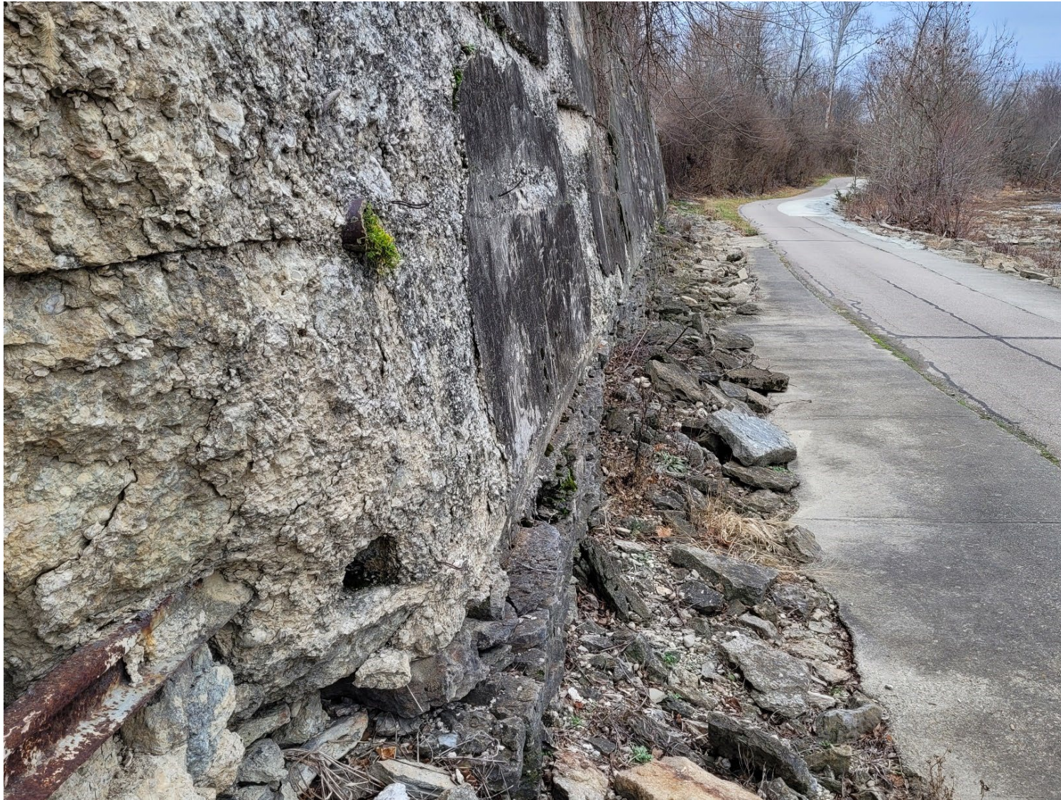
Figure 5: Dayton Cincinnati Pike – South Wall Section Showing Original Batter
