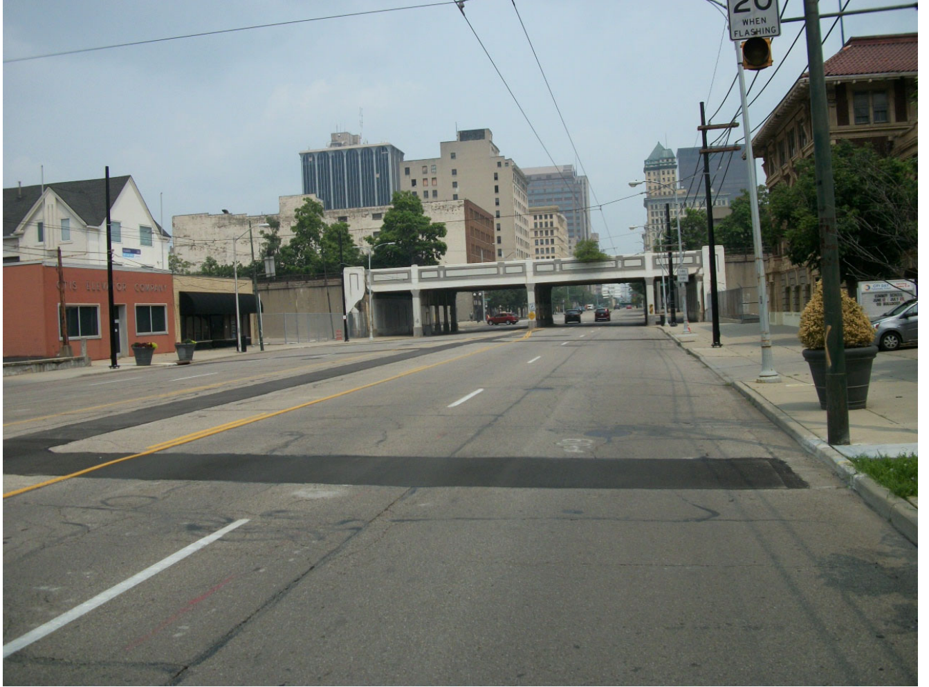
Northbound Main South of Sixth Street
