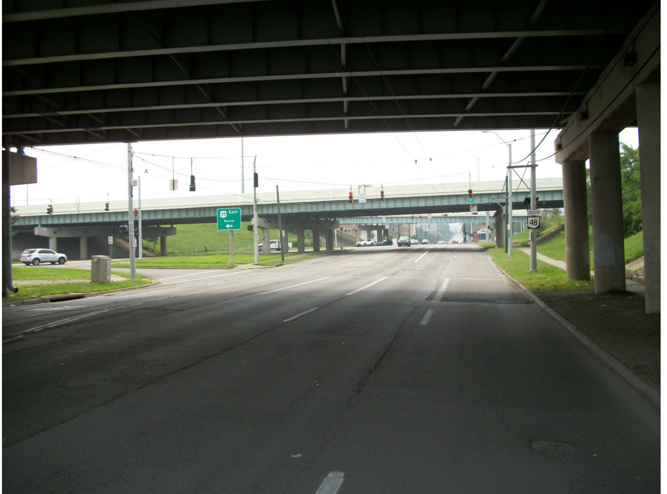
Southbound Main at US 35 Ramp
