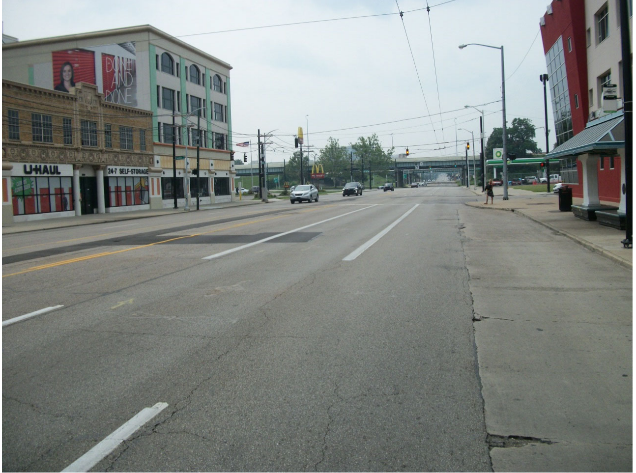
Southbound Main North of Franklin
