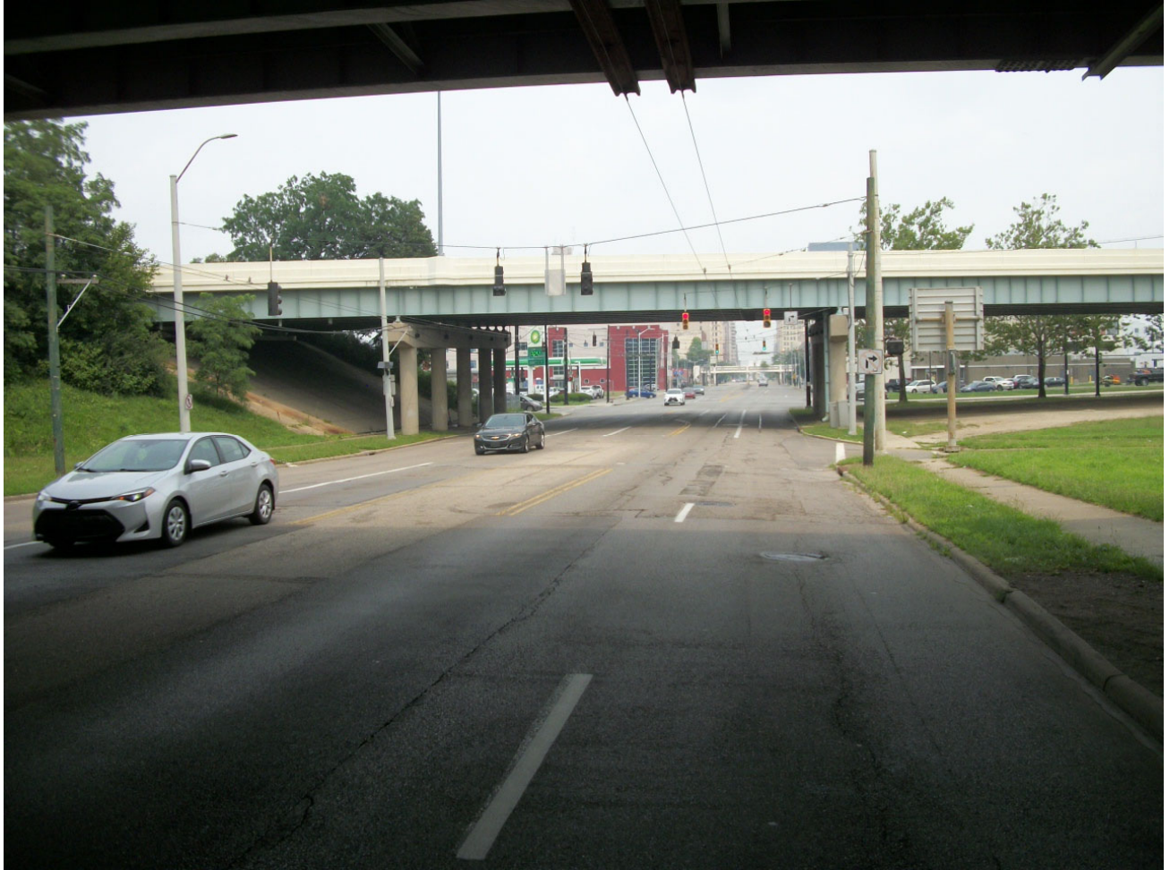
Northbound Main South of US 35 Ramp
