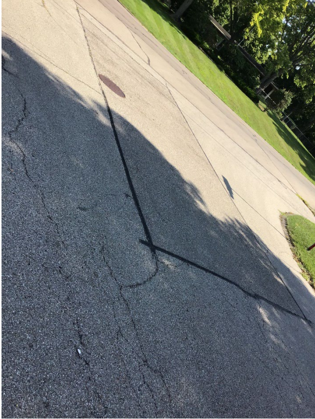
Silbury Lane patch, facing north
