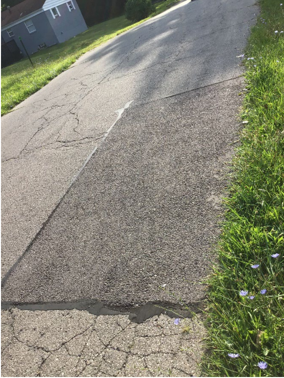
Natchez Ave patch, facing east
