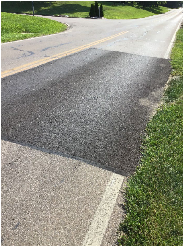
Rahn Road patch, facing east
