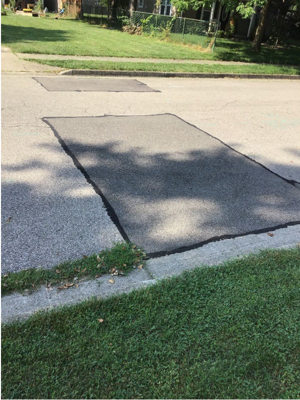
Eldorado Ave patches, facing west
