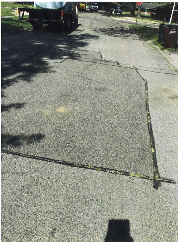
Frieda Ln patch, facing northwest
