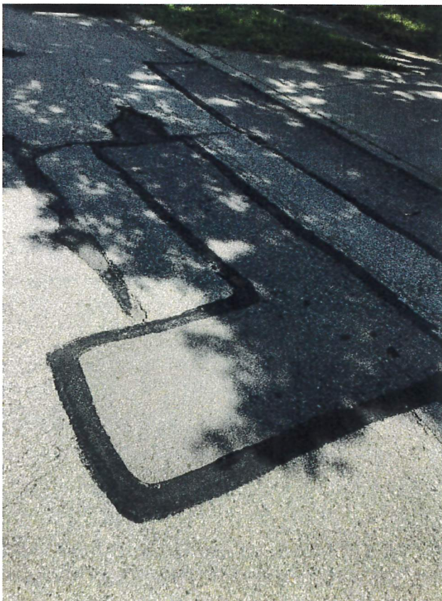
Sunray Rd patches, facing north
