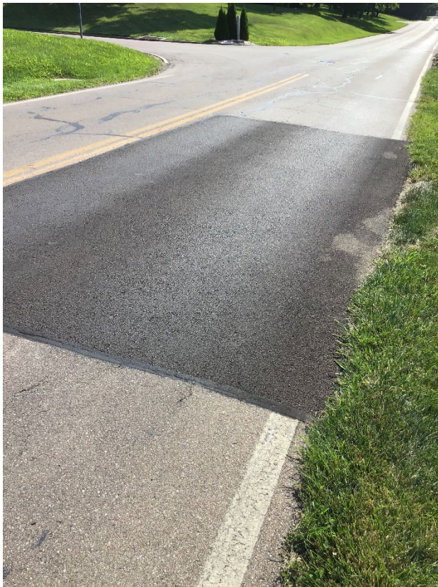
Rahn Road patch, facing east
