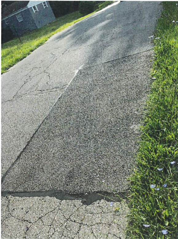
Natchez Ave patch, facing east
