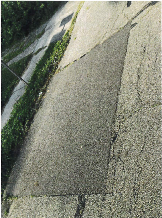
Natchez Ave patch, facing east
