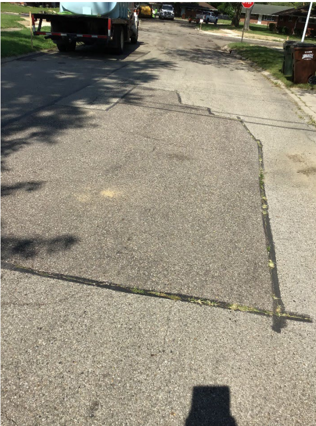
Frieda Ln patch, facing northwest
