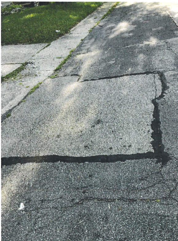
Nevada Ave patch, facing east
