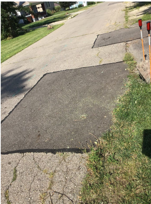
Dexter Ave patches, facing west
