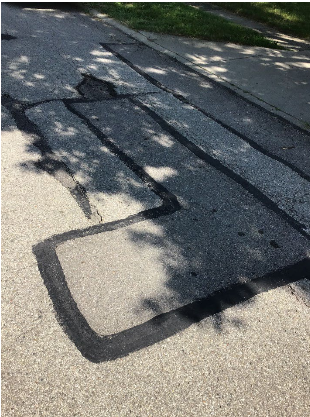
Sunray Rd patches, facing north
