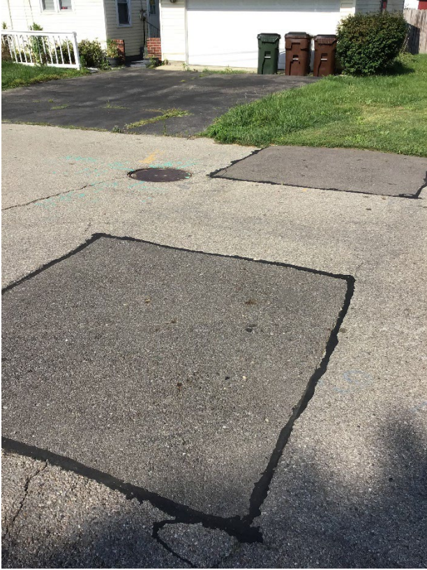
Dexter Ave patches, facing west
