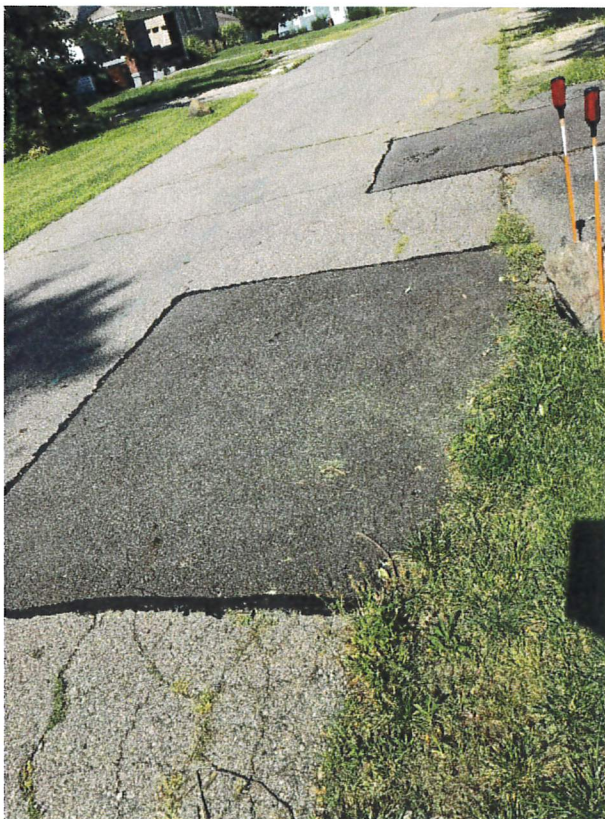
Dexter Ave patches, facing west
