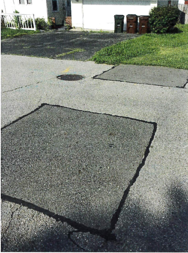
Dexter Ave patches, facing west
