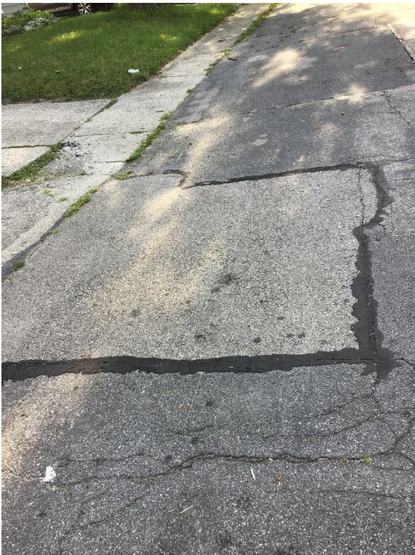
Nevada Ave patch, facing east
