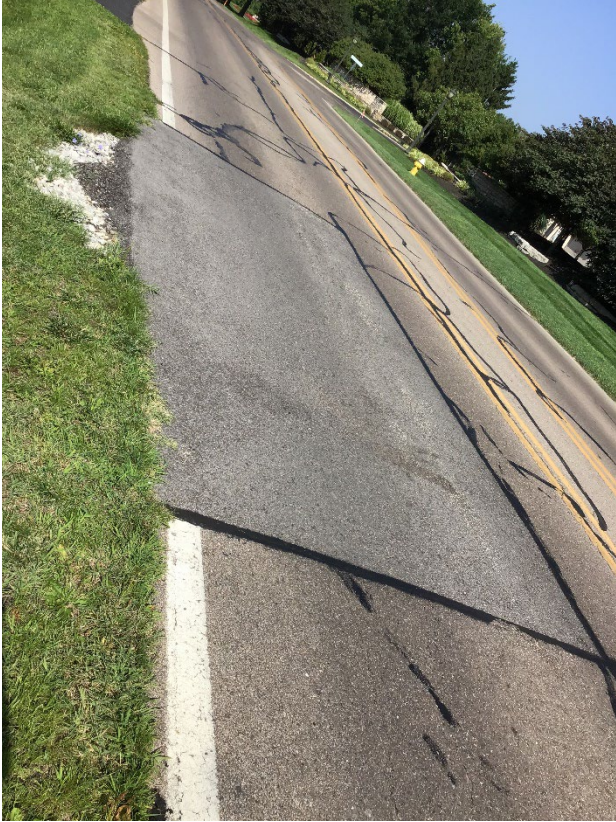
Rahn Road patch, facing east
