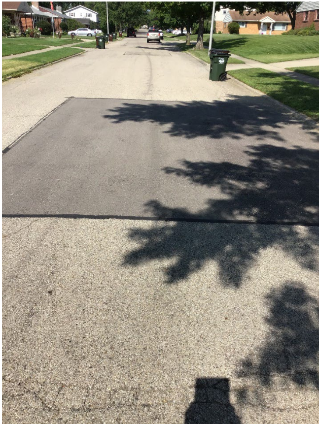
Rio Ln patch, facing west
