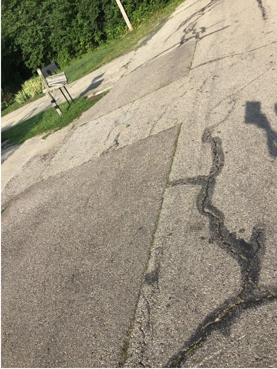
Annapolis Ave patches, facing west Natchez, Annapolis, Nevada WMR Project
