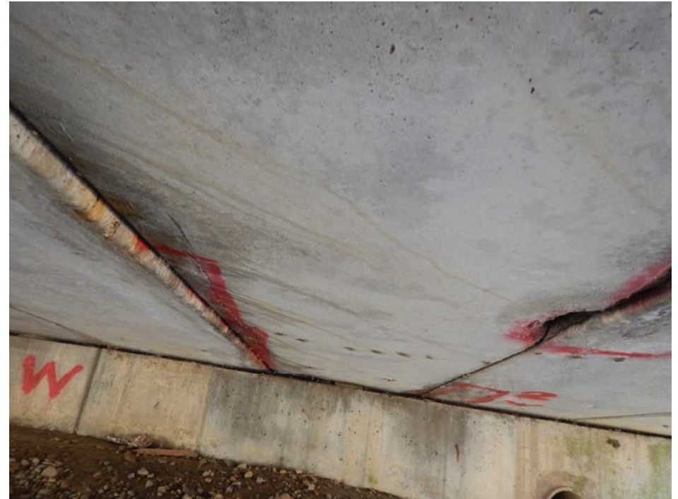
Beam 3 Looking West
