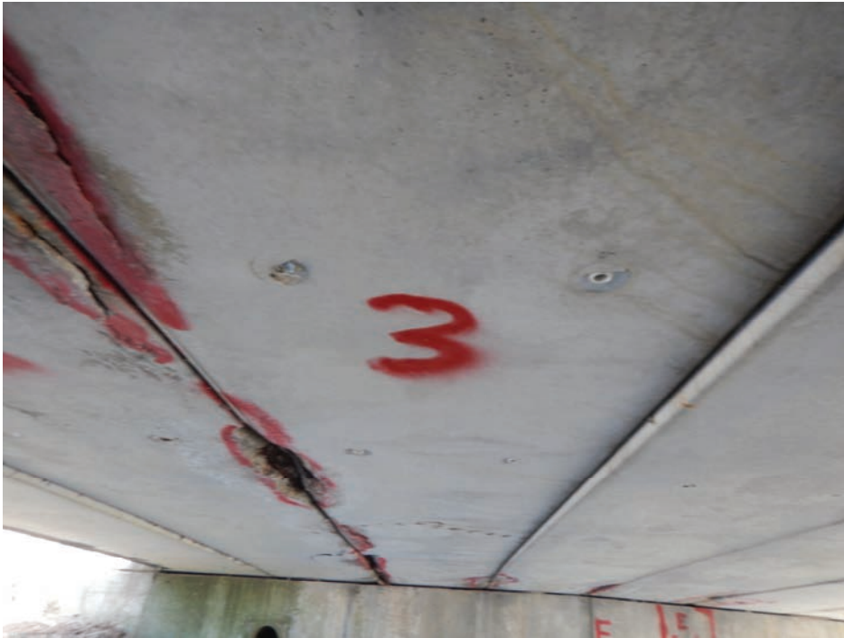
Beam 3 Looking East
