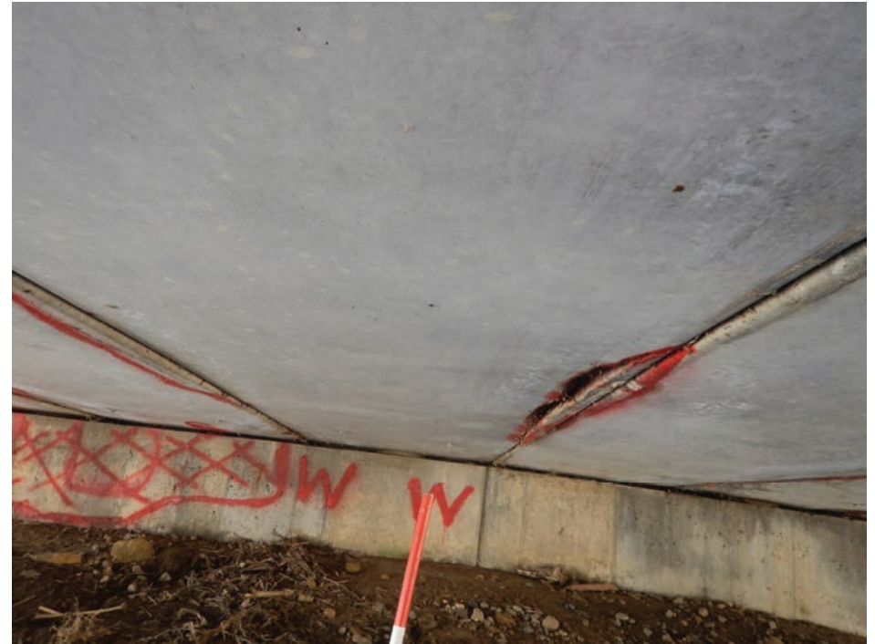
Beam 5 Looking West
