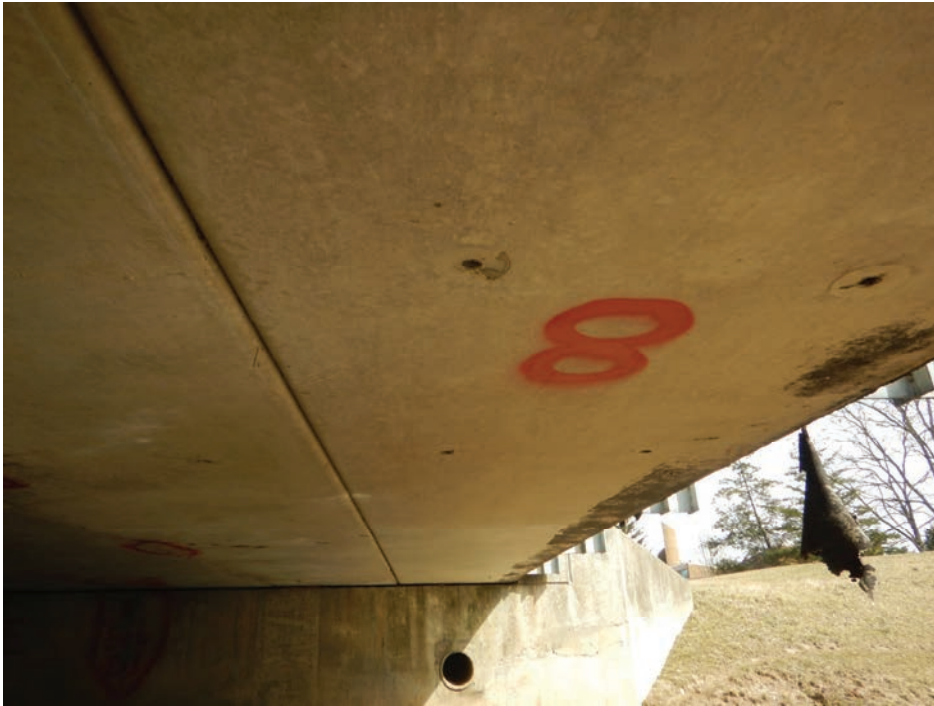
Beam 8 Looking East
