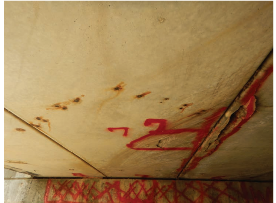
Beam 7 Looking West
