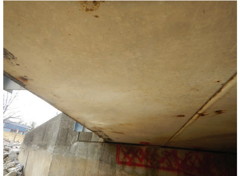
Beam 8 Looking West
