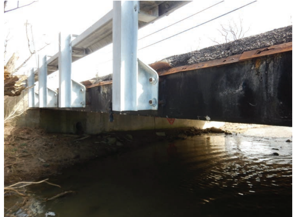
North Deck Drainage
