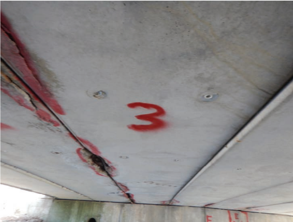
Beam 3 Looking East
