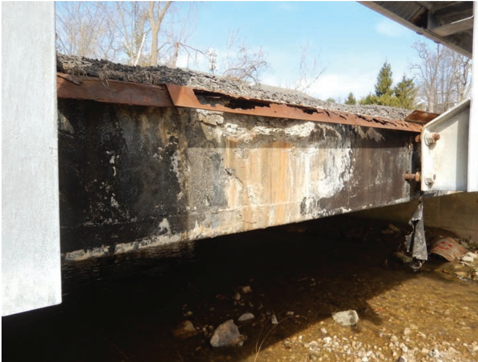
South Deck Drainage
