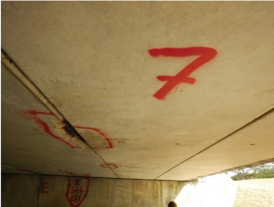
Beam 7 Looking East
