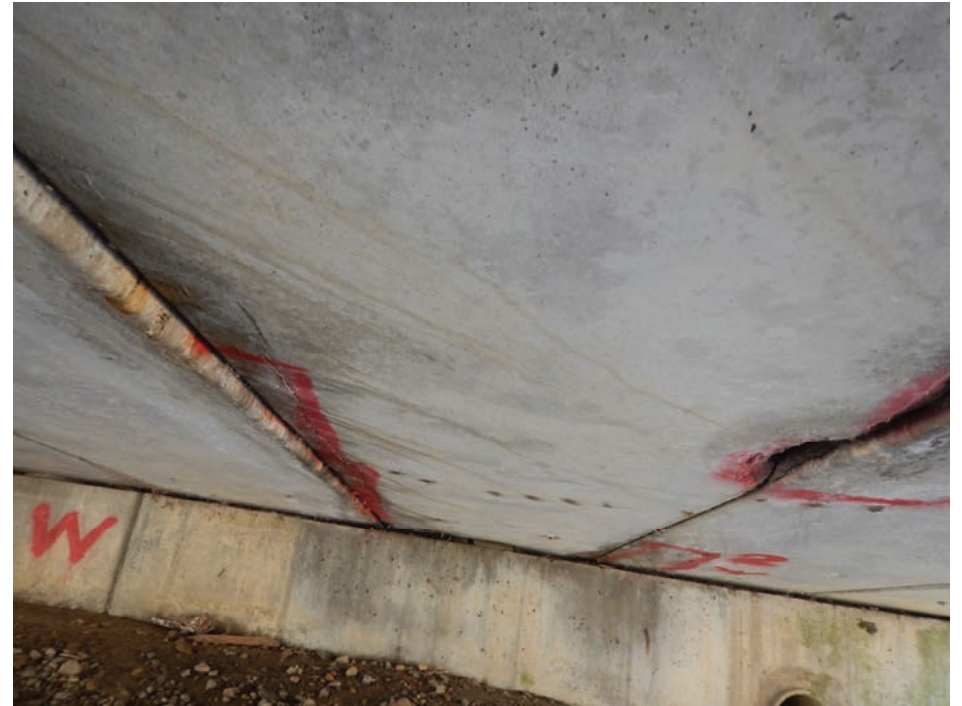
Beam 3 Looking West
