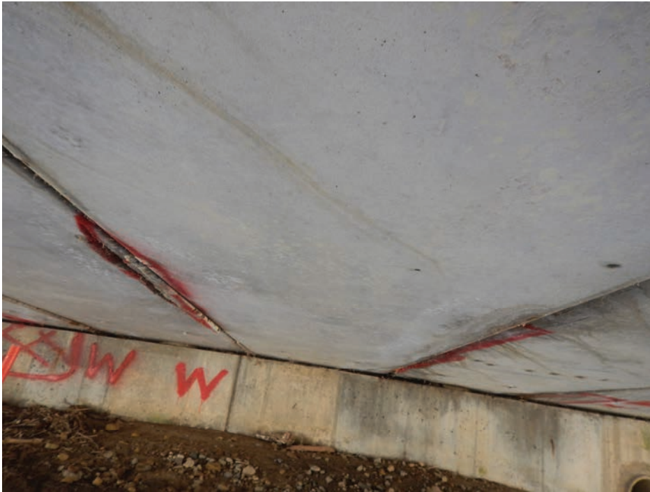
Beam 4 Looking West
