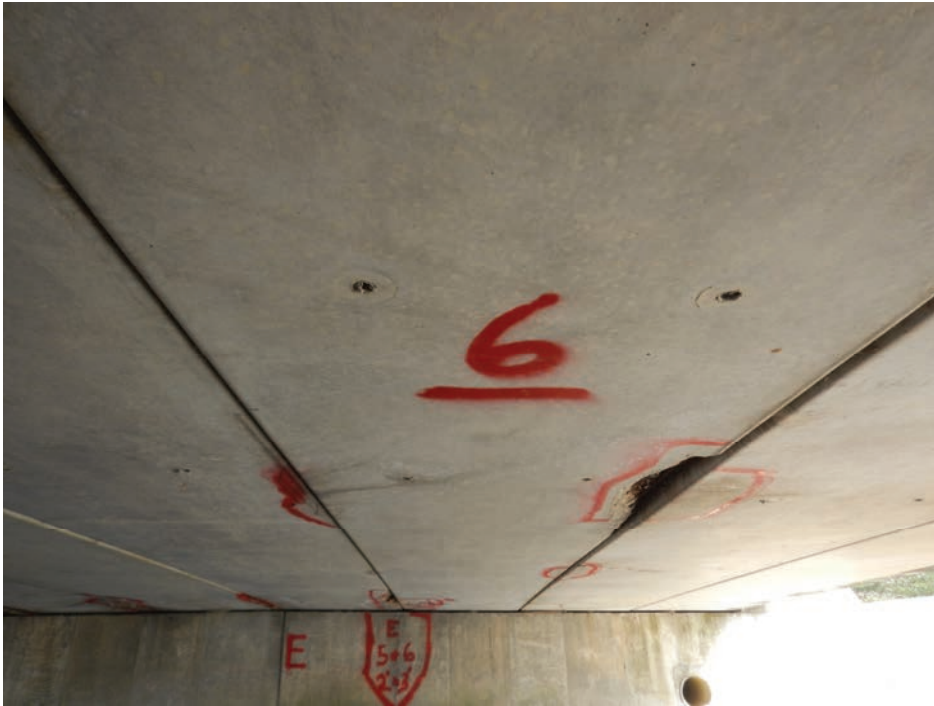
Beam 6 Looking East
