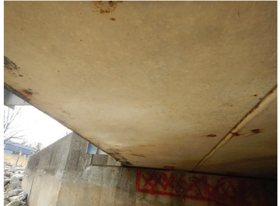
Beam 8 Looking West
