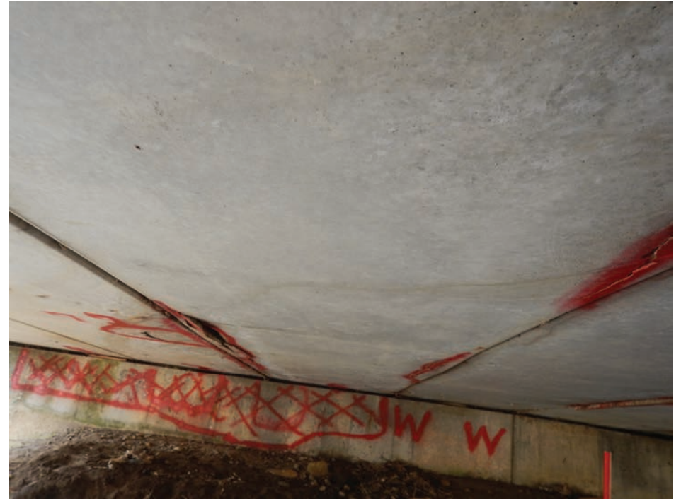
Beam 6 Looking West
