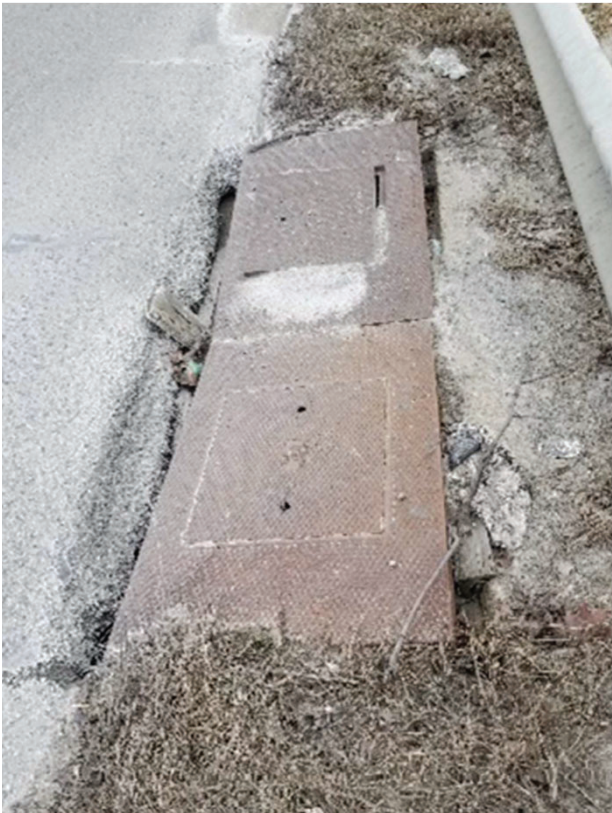
Southwest Drainage Inlet
