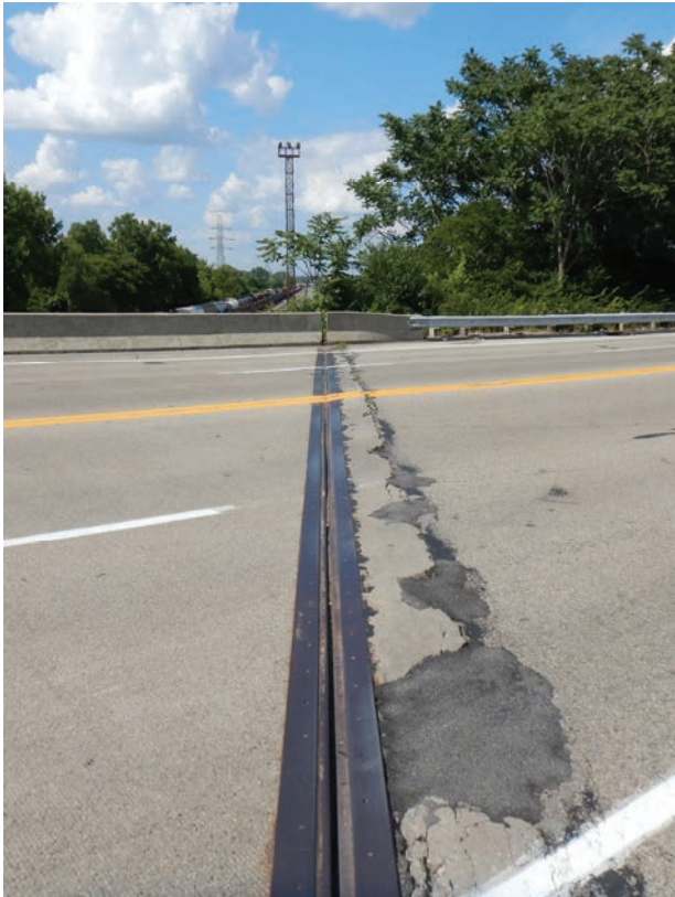
East/Forward Expansion Joint
