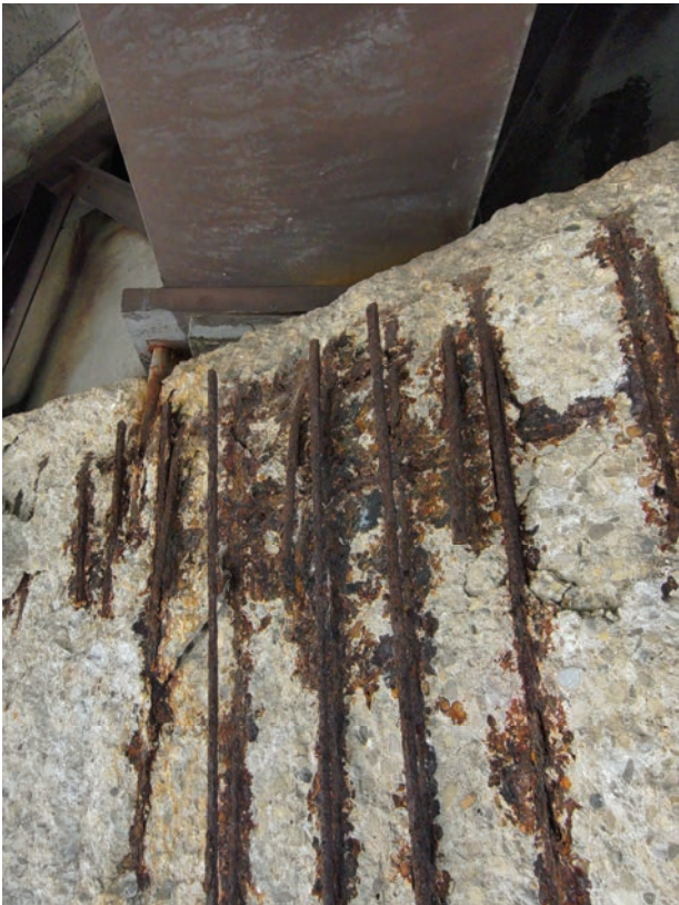
West/Rear Beam Seat Showing the Exposed Anchor Rod and Loss of Bearing Area Beneath Beam-2
