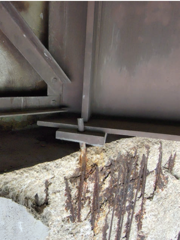
West/Rear Beam Seat Showing the Exposed Anchor Rod and Loss of Bearing Area Beneath Beam-2
