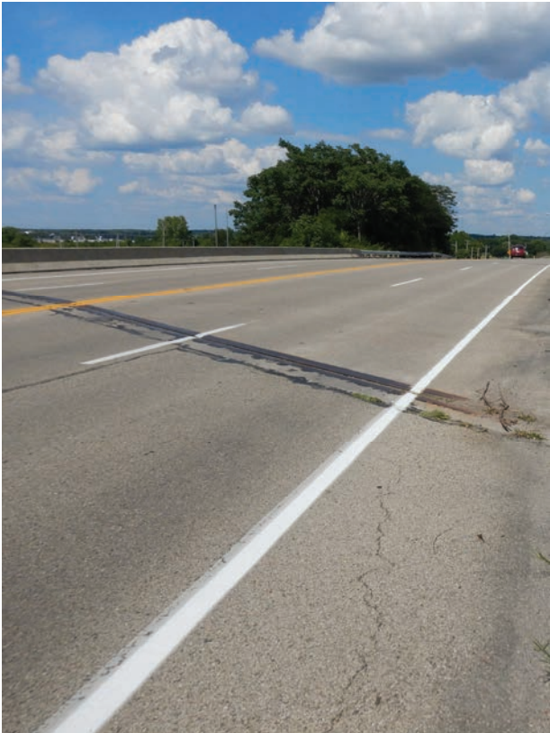
West/Rear Expansion Joint
