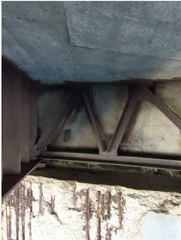
West/Rear Beam Seat Showing the Exposed Anchor Rod and Loss of Bearing Area Beneath Beam-2
