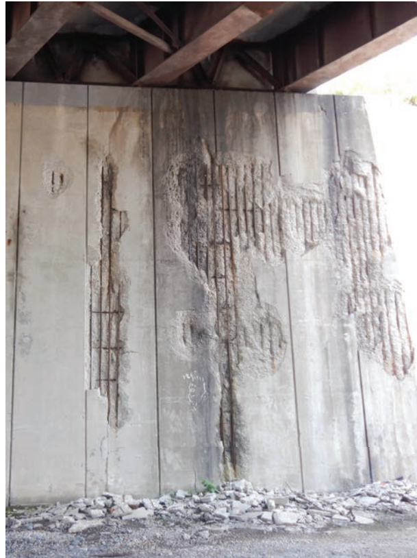
East/Forward Abutment Wall
