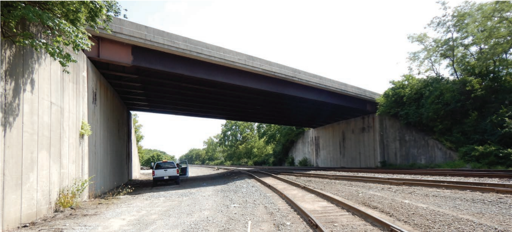
Profile View of the Wagner Ford Road Bridge over the CSX Railroad as seen from the North Looking South
