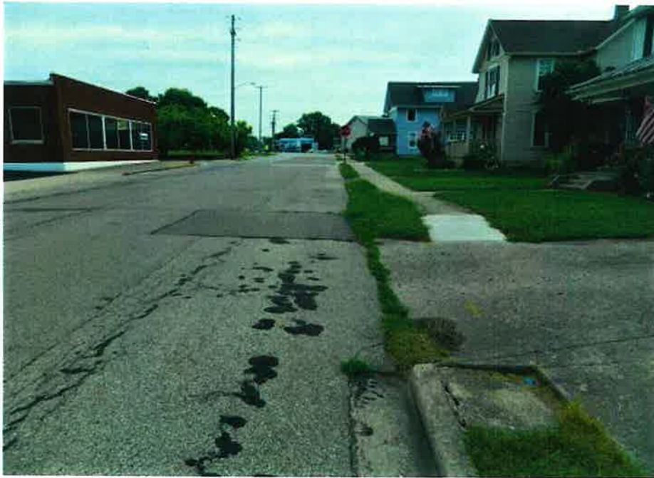
Hay Avenue, Phase 2 – Current Roadway Conditions
