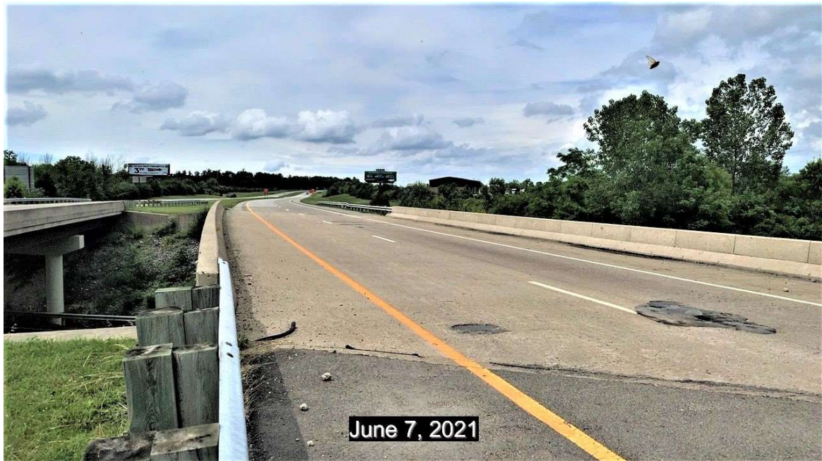
PHOTO 2 Condition Description End view looking north.
