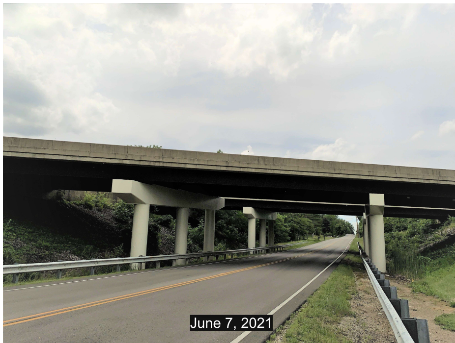
PHOTO 4 Condition Description East fascia looking west.
