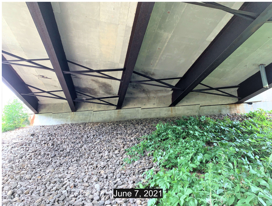
PHOTO 9 Condition Description Looking at north Abutment Wall, Span 3.
