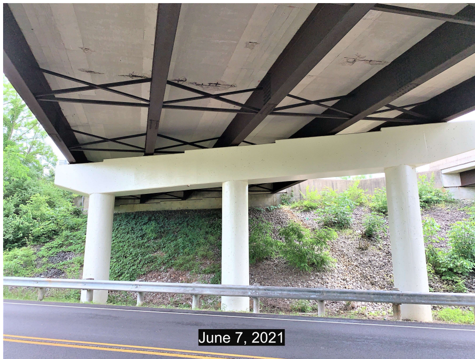
PHOTO 6 Condition Description Looking at north face of pier 1, span 2.
