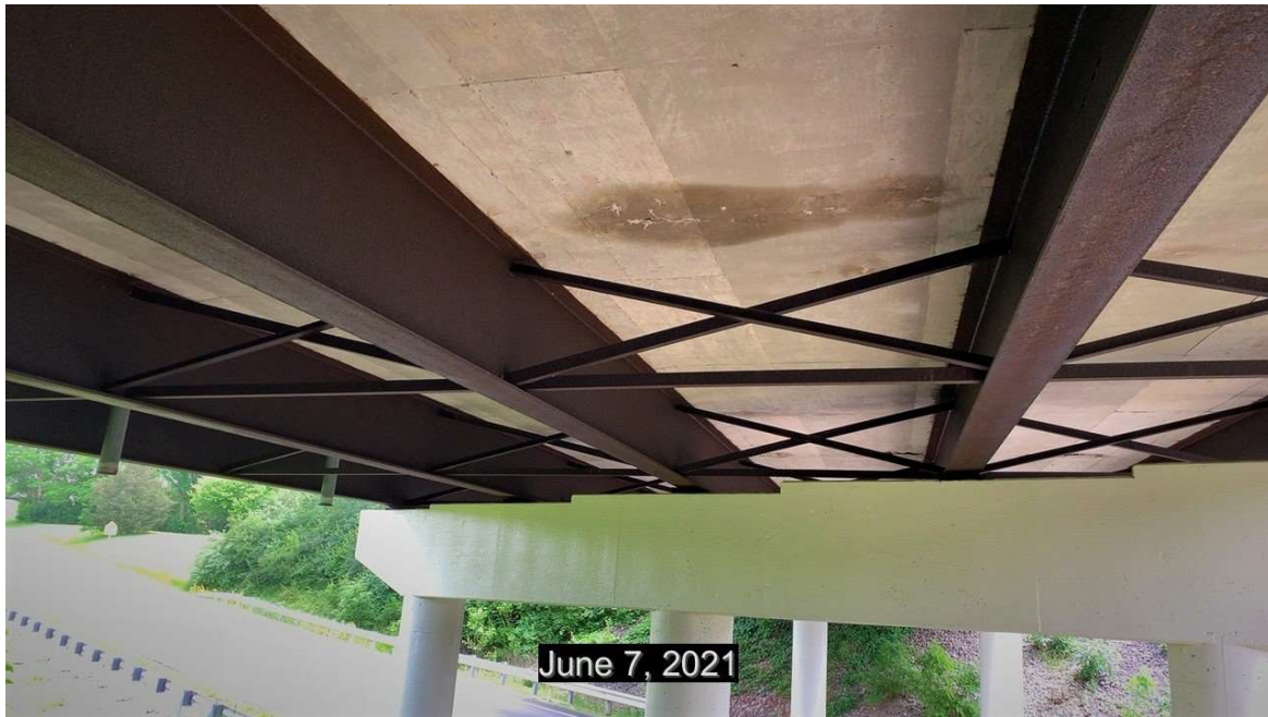
PHOTO 8 Condition Description Looking at north face of Pier 2, Span 3.
