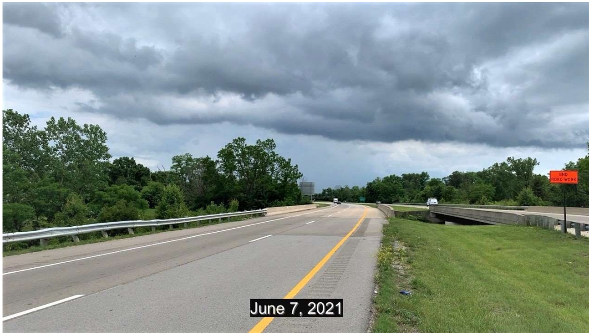
PHOTO 1 Condition Description End view looking south.
