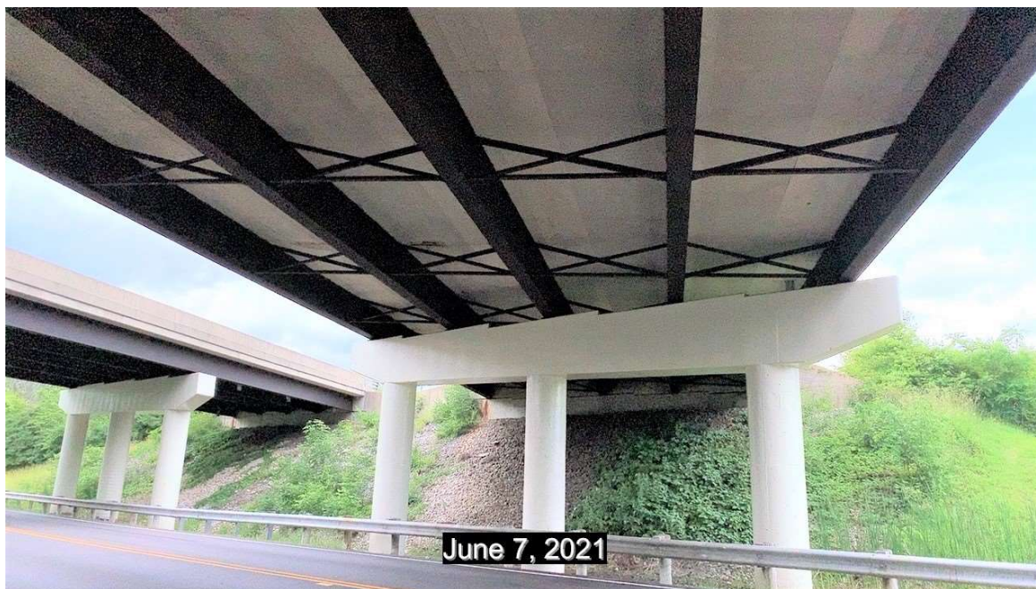
PHOTO 7 Description Looking at south face Pier 2, Span 2.
