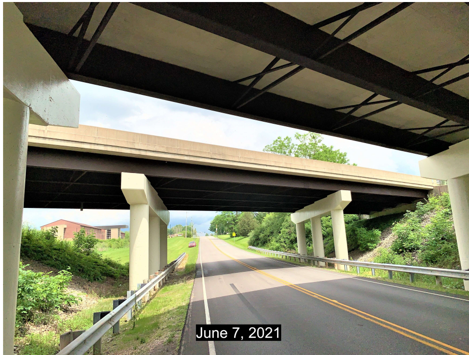
PHOTO 3 Condition Description West fascia looking east.
