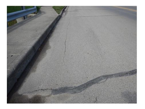
Discoloration of concrete; lots of interior moisture in the beams; shear key damage between the beams; top of abutment cracked; exposed reinforcing steel
