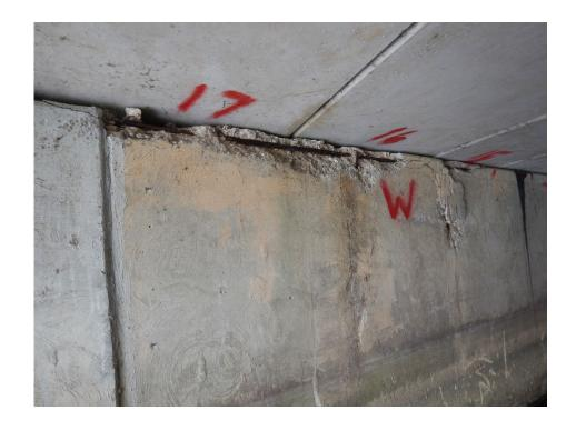
Some areas on the abutment wall have a major crack towards the top edge. The bridge is posted at 15 tons for 2 axle trucks.
