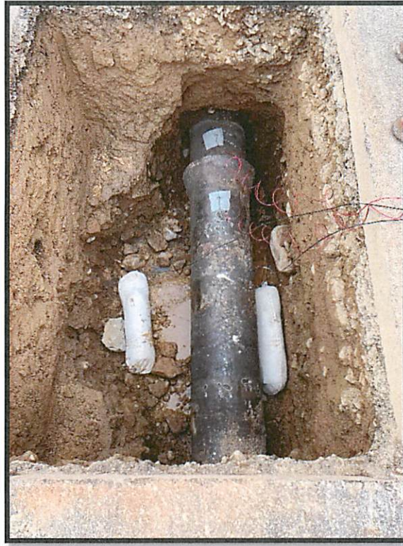
Two 32# anodes installed at Dig 3
