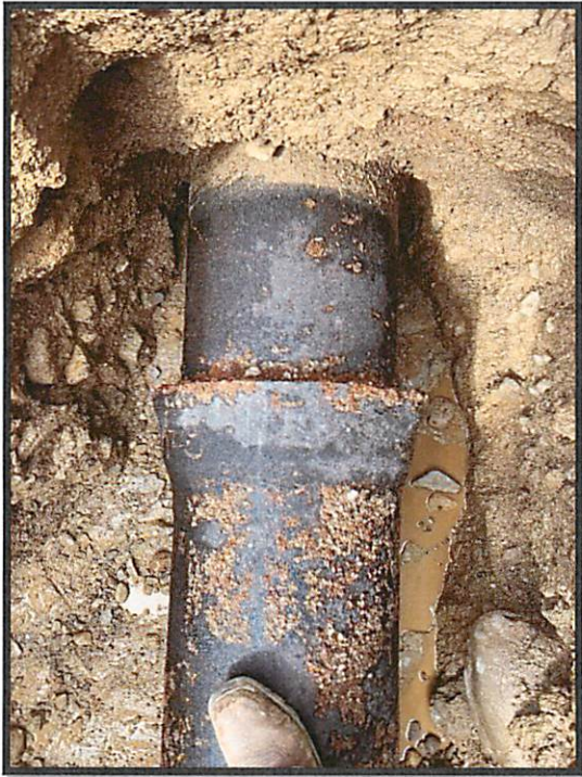
Joint at Dig 3
