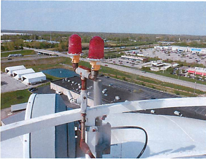
25) The double aviation light appears to be in good condition.
