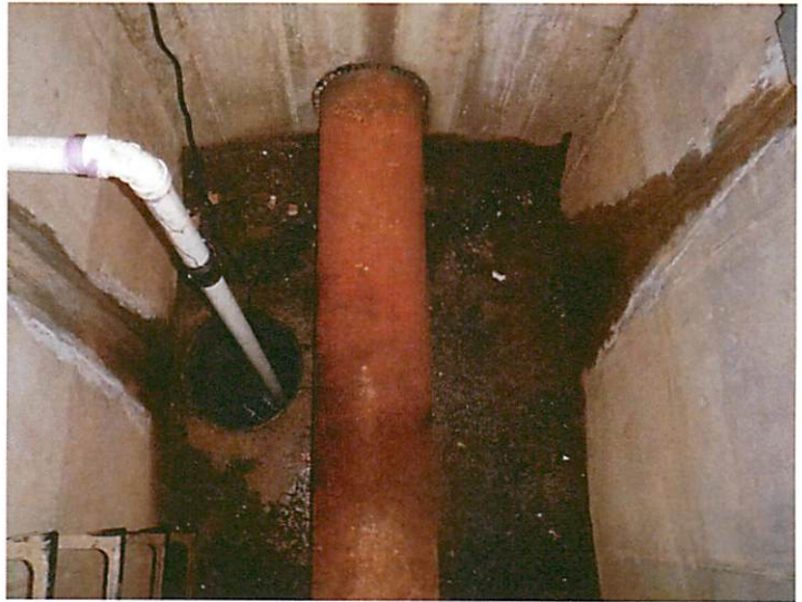
74) The coating on the pit piping is in fair condition.
