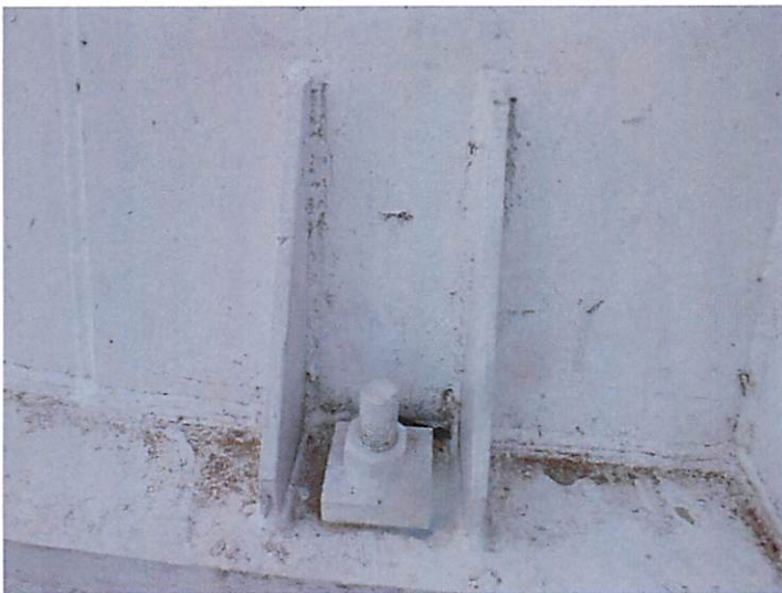
3) The basebell anchor bolts are in good condition.
