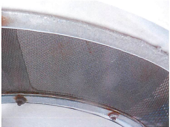
32) The screened pressure plate was found to be in good condition.
