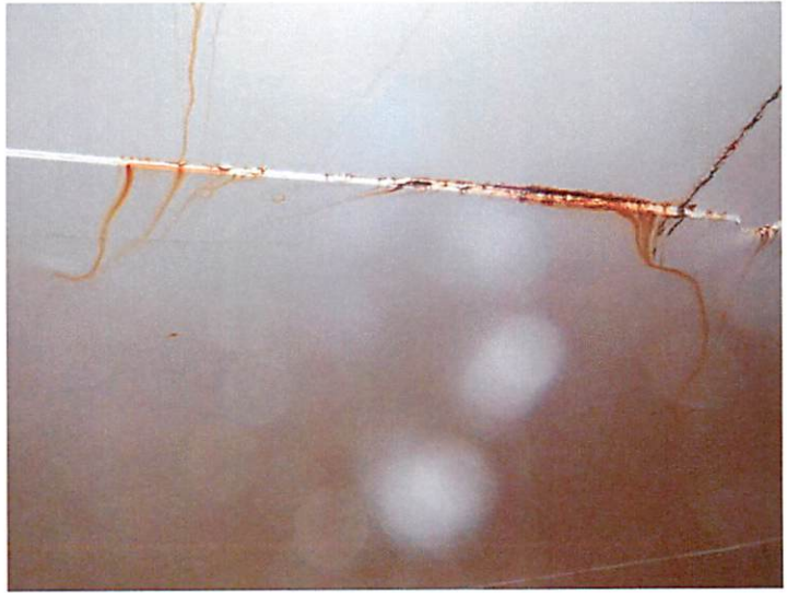
59) The wet interior roof coating is in good condition.
