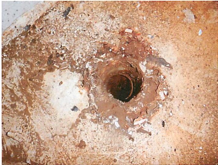
44) The condensate platform drain appears to be in good condition.
