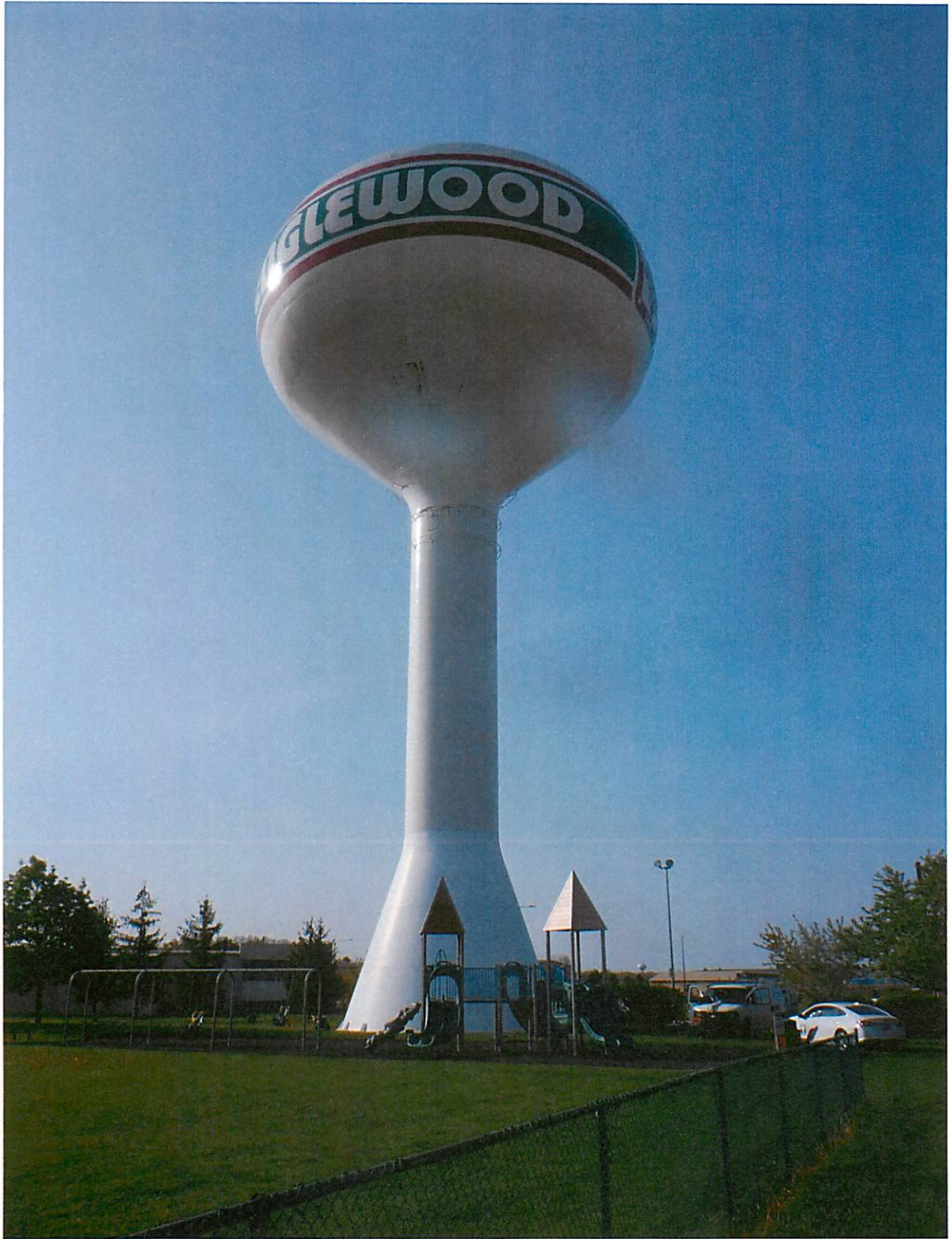
1,000,000 gallon spheroid (South) located in Englewood, Ohio
