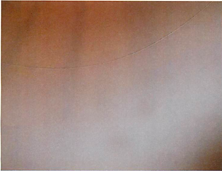
46) The coating in the riser is in good condition.
