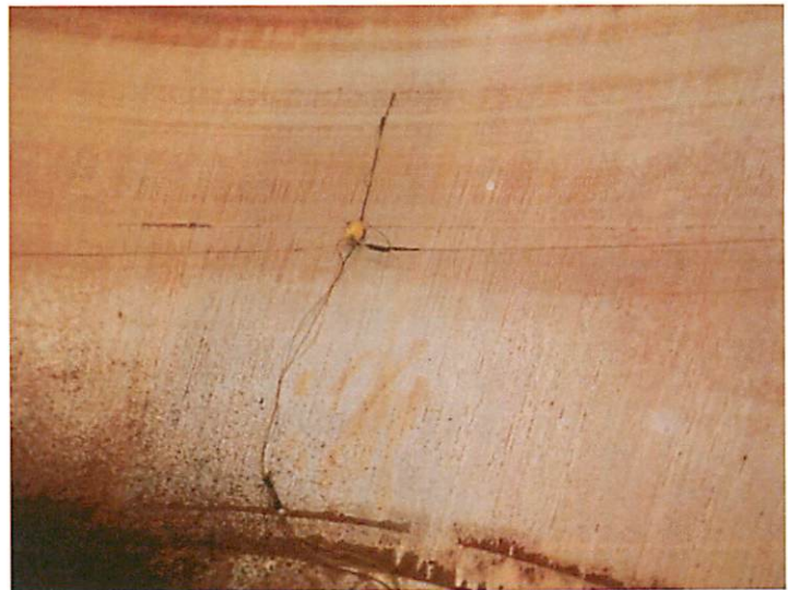
68) The cathodic protection system appears to be in good condition.
