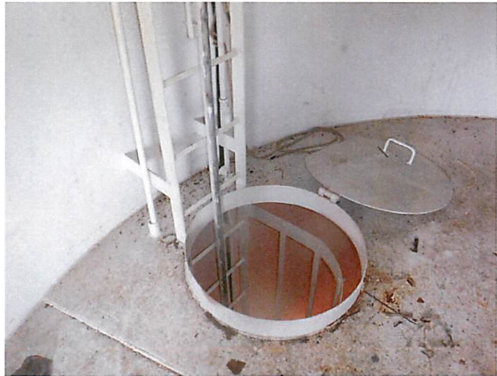
47) The top platform opening is equipped with a hinged cover.
