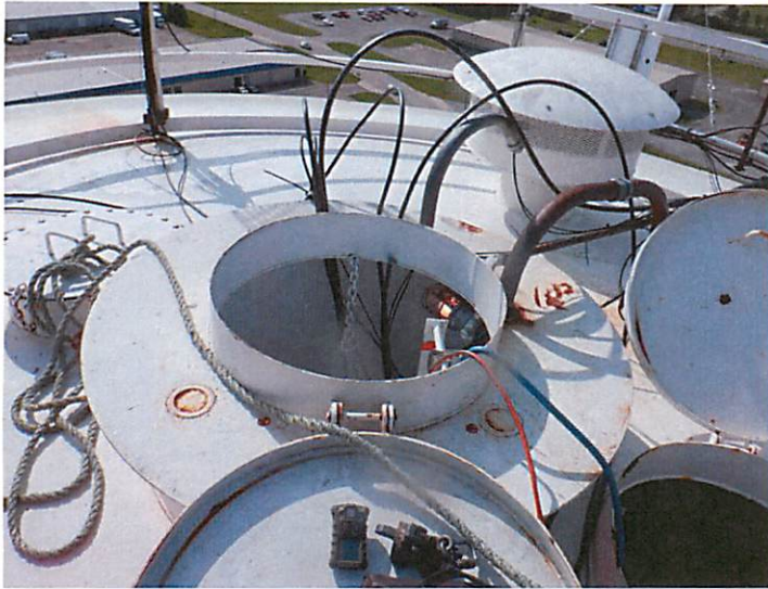
19) The dry interior hatch is in good condition.
