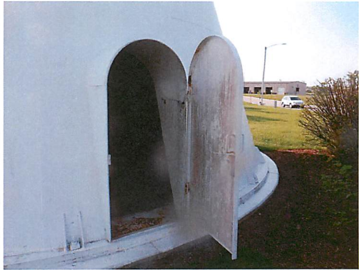
5) The service door operated properly during the inspection.
