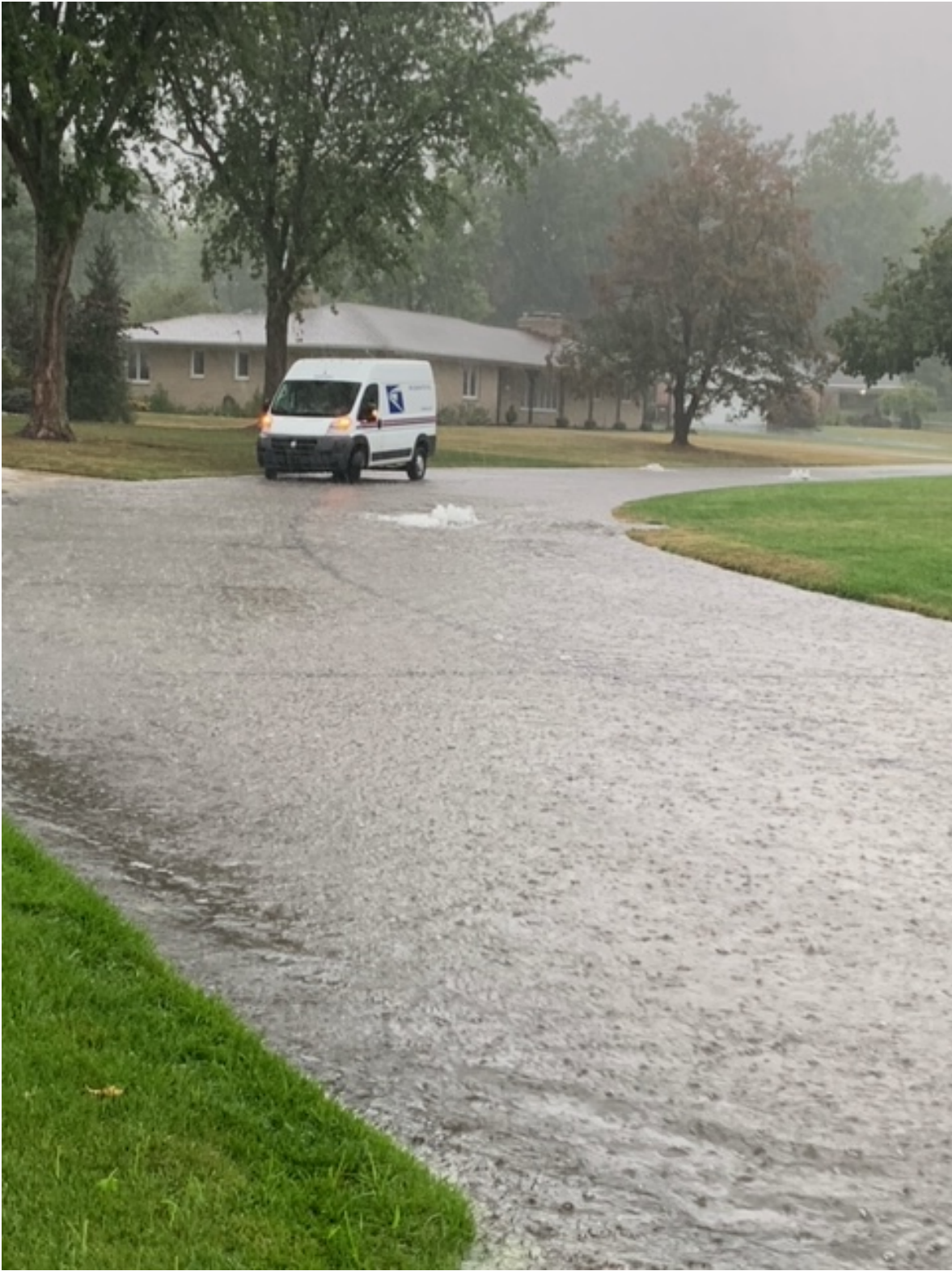
Street Flooding and multiple drainage structures surcharging at location #1
