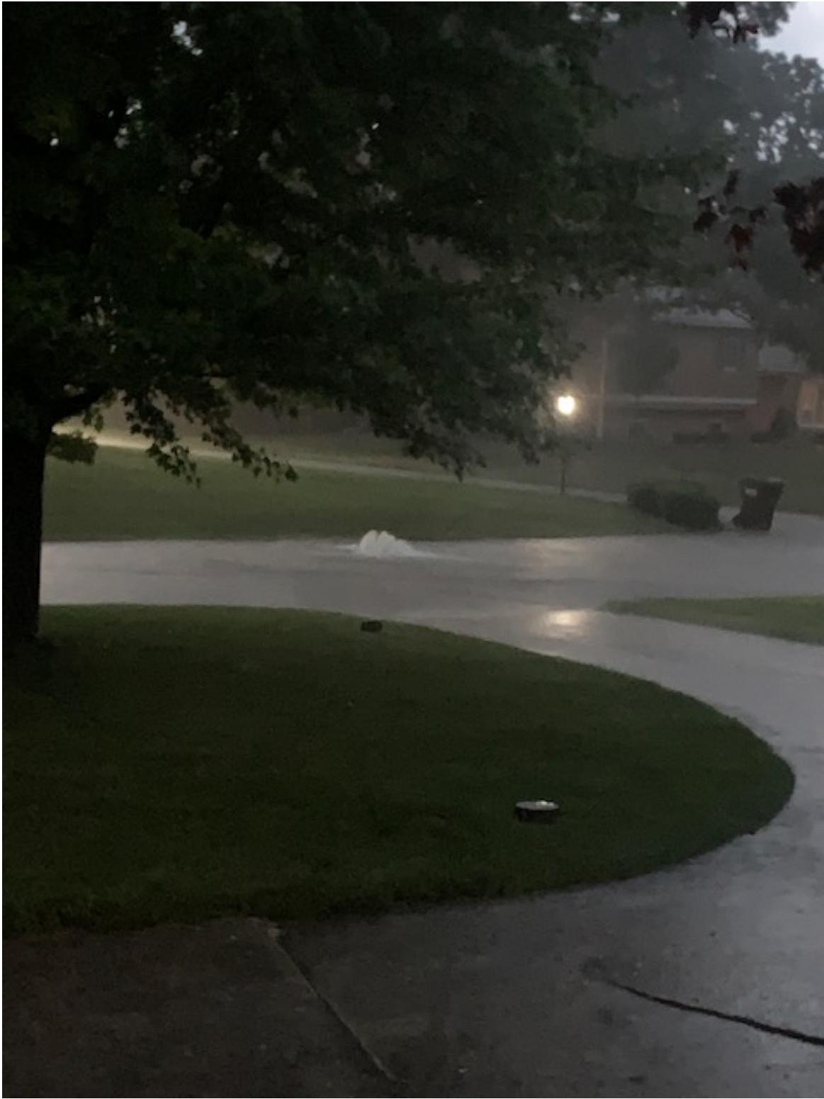
Street Flooding and manhole surcharging at location #1
