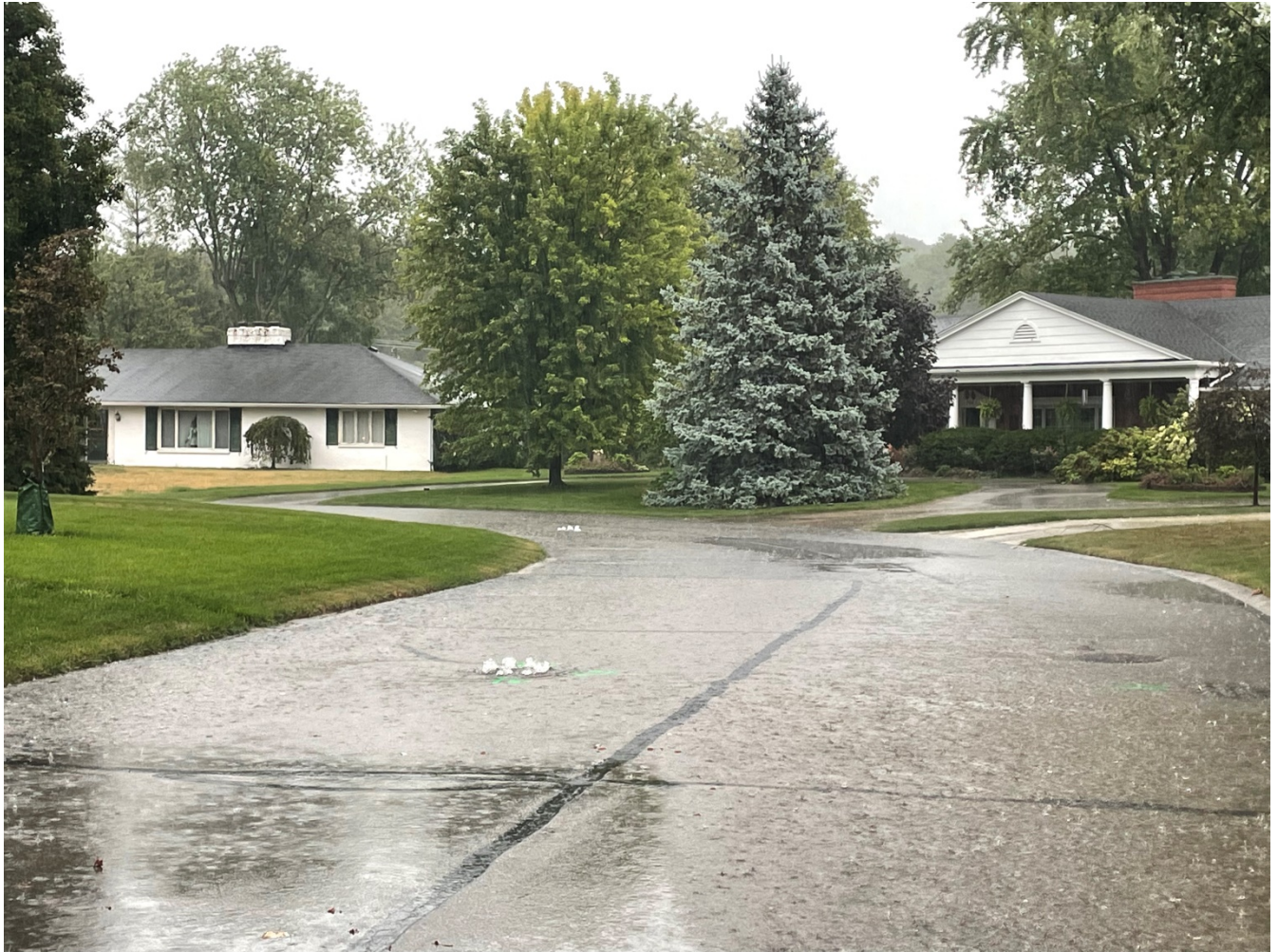
Street Flooding and multiple drainage structures surcharging at location #2
