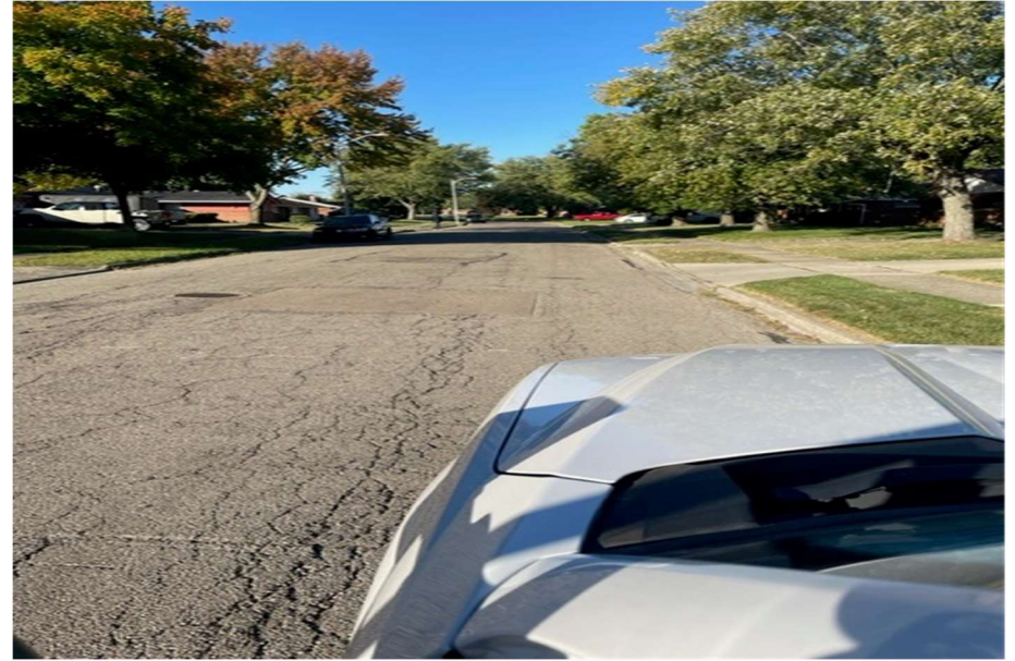
800 MacMillan Drive (1 Water Main Break)
