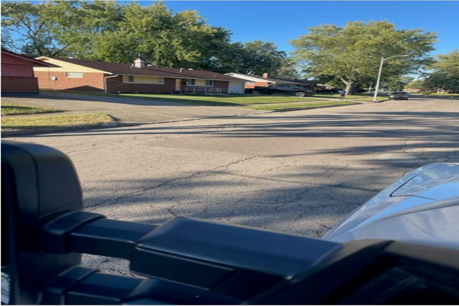
816 MacMillan Drive (1 Water Main Break)
