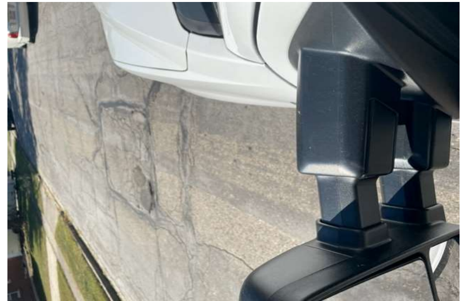
629 N. Eppington Drive (1 Water Main Break)
