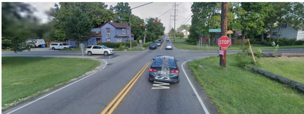
PHOTO 1: EB SIEBENTHALER AVENUE APPROACH TO CATALPA DR
